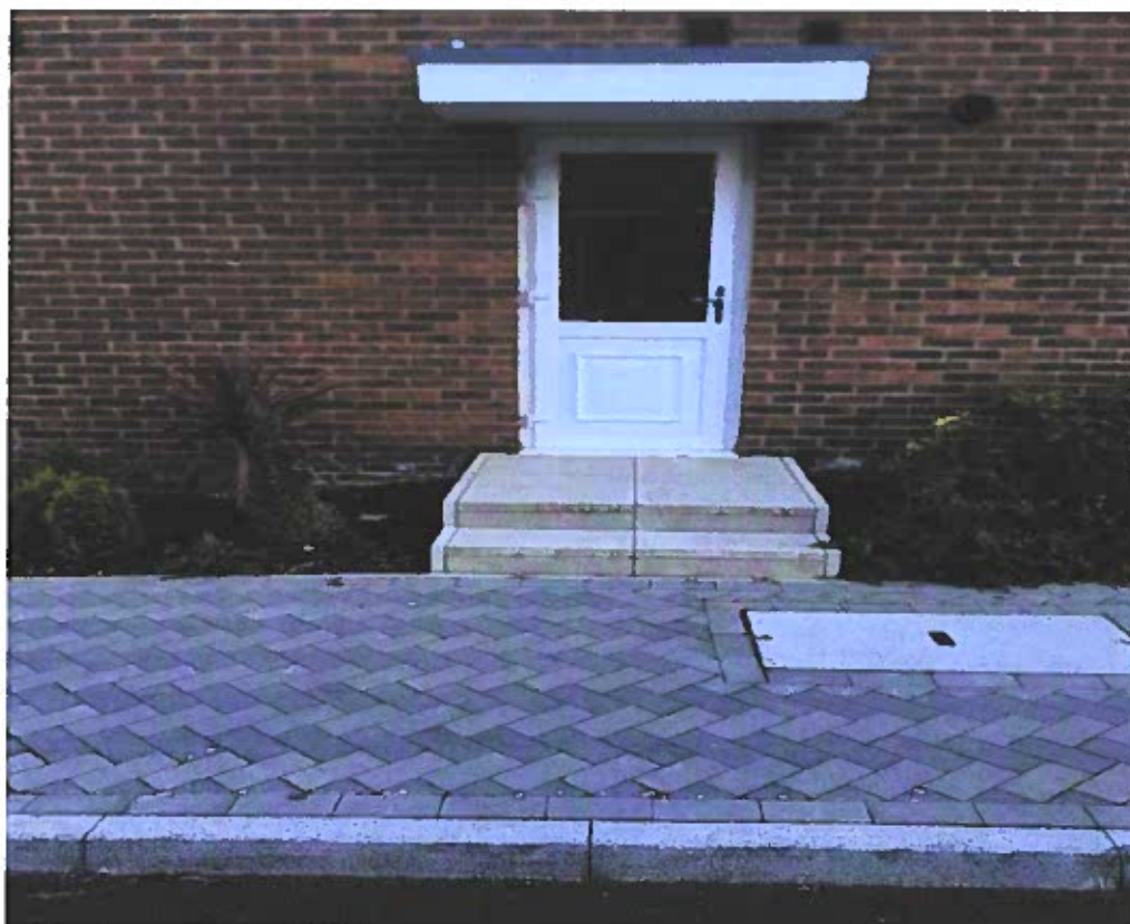
Figure 2 (above): Utility Room Door
