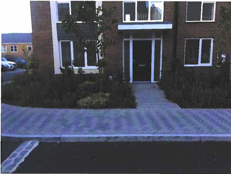
Figure 1 (above): Front Door
