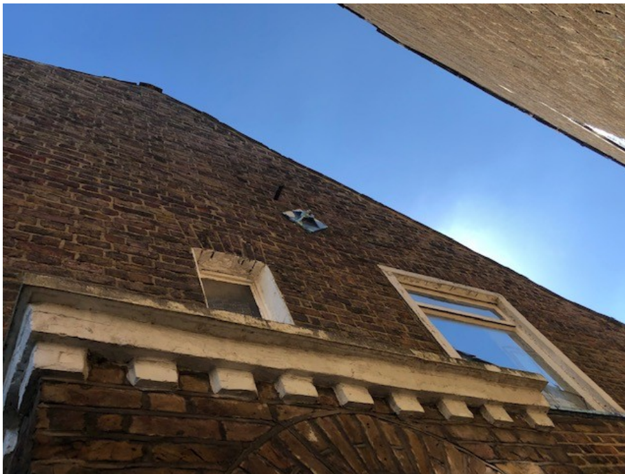
Fig. 15. The windows in the side elevation (photo provided by Jordan Wang).
