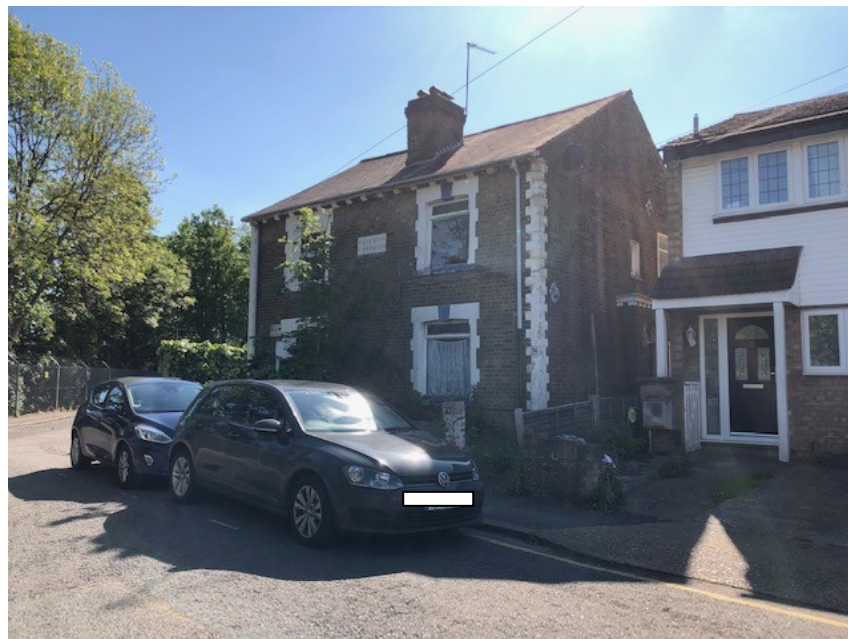
6.2 The house is accessed via the main entrance door in the side alley (Fig. 12), via a projecting brick doorway with dentil moulded flat roof which has a replacement door with segmental arch above (Fig. 13). The alley also gives access to the rear garden through a wooden gate on the west side of the property (Fig. 14).
