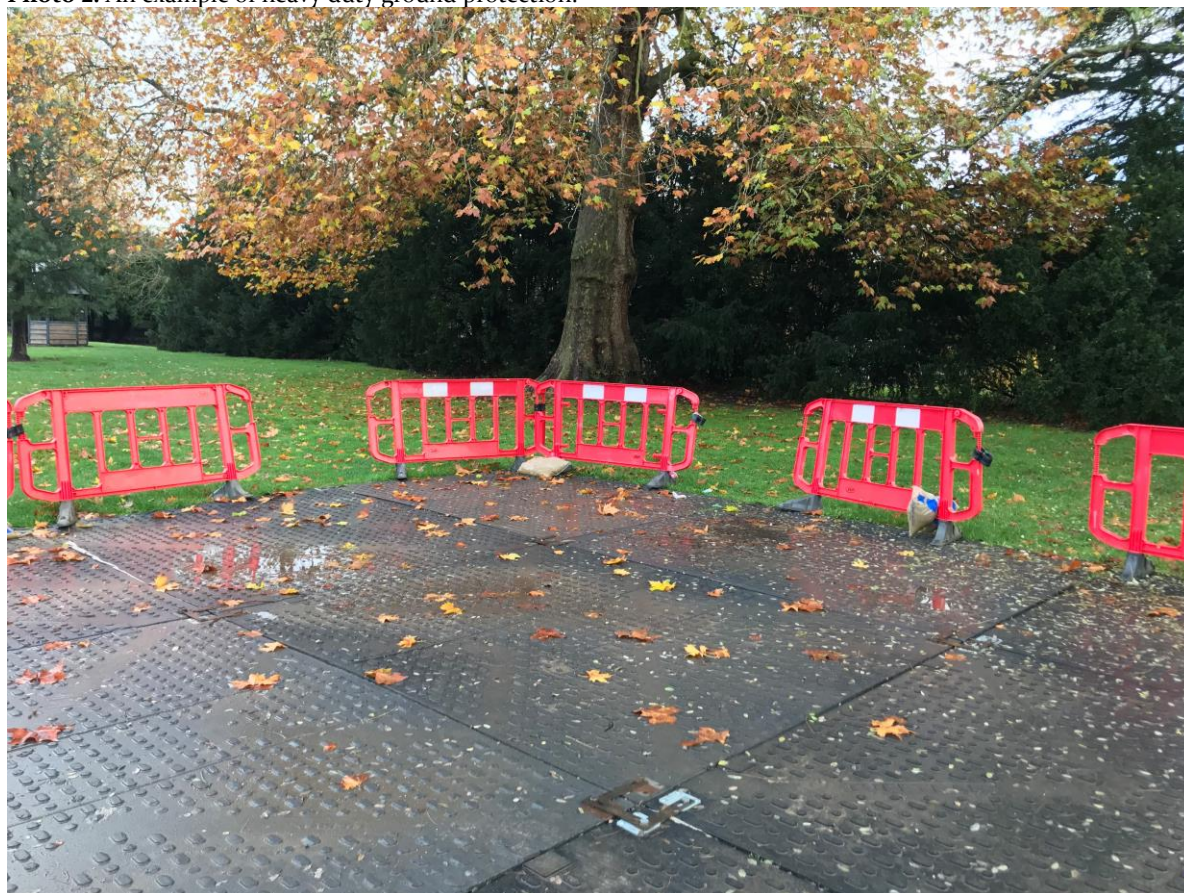
Photo 2. An example of heavy duty ground protection.
