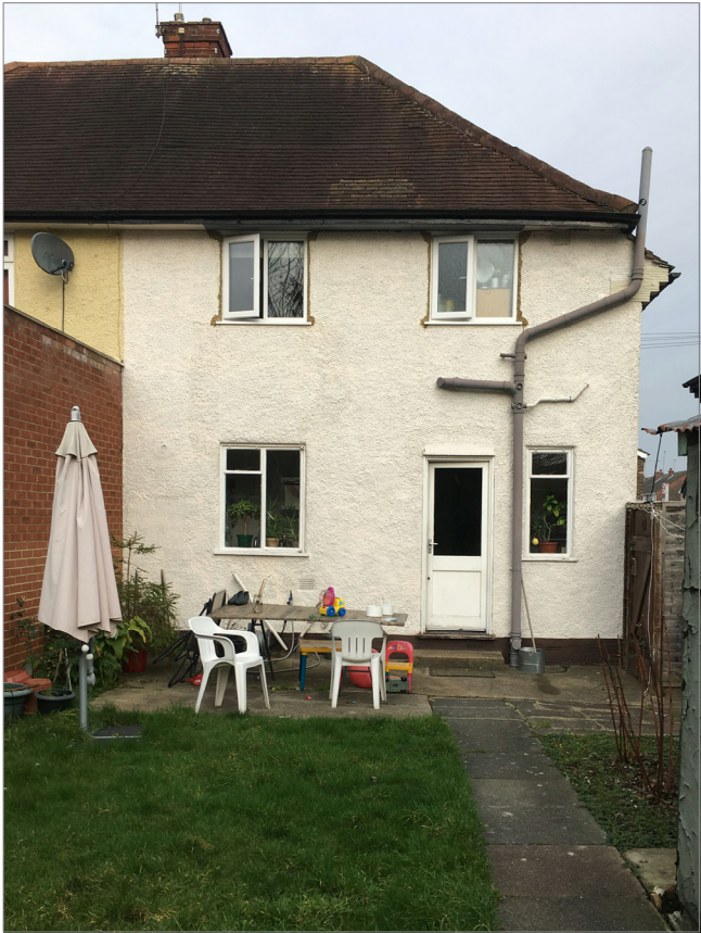
Site Photo Rear Facade
