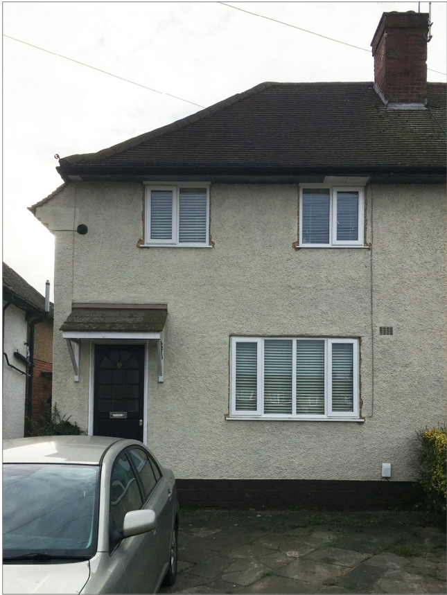
Site Photo Front Facade
