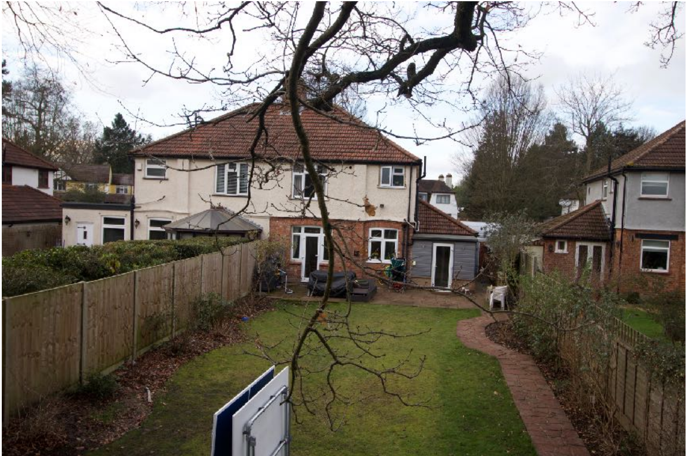
Rear elevation facing view
