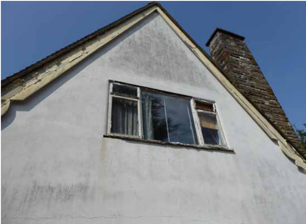
Existing facade close-up
