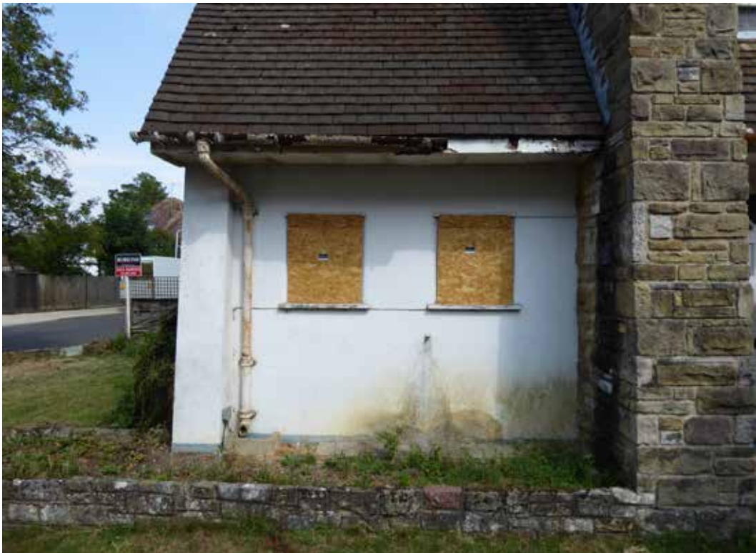
Existing facade close-up
