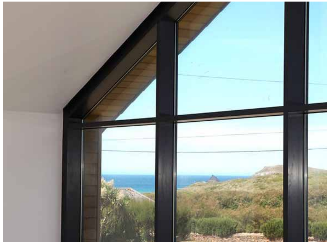
Glazed Gable End South Facade Wall
