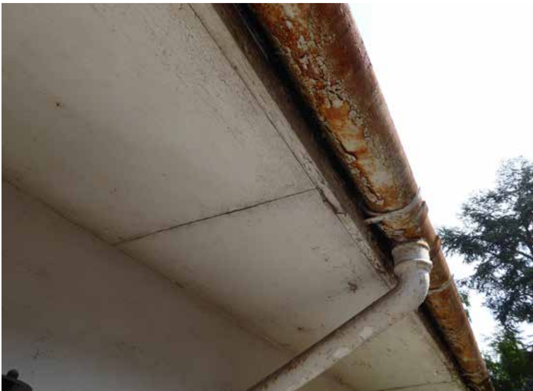
Painted Cast Iron Gutters
