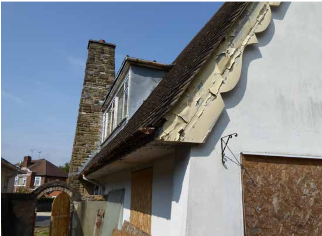
Painted Timber Soffit Facia and Barge Board
