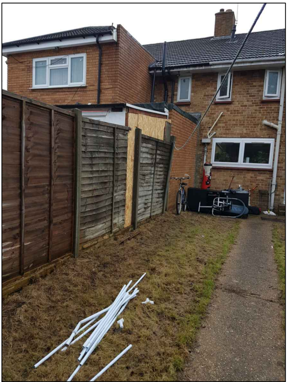
VIEW OF REAR ELEVATION NO 29 AND 31
