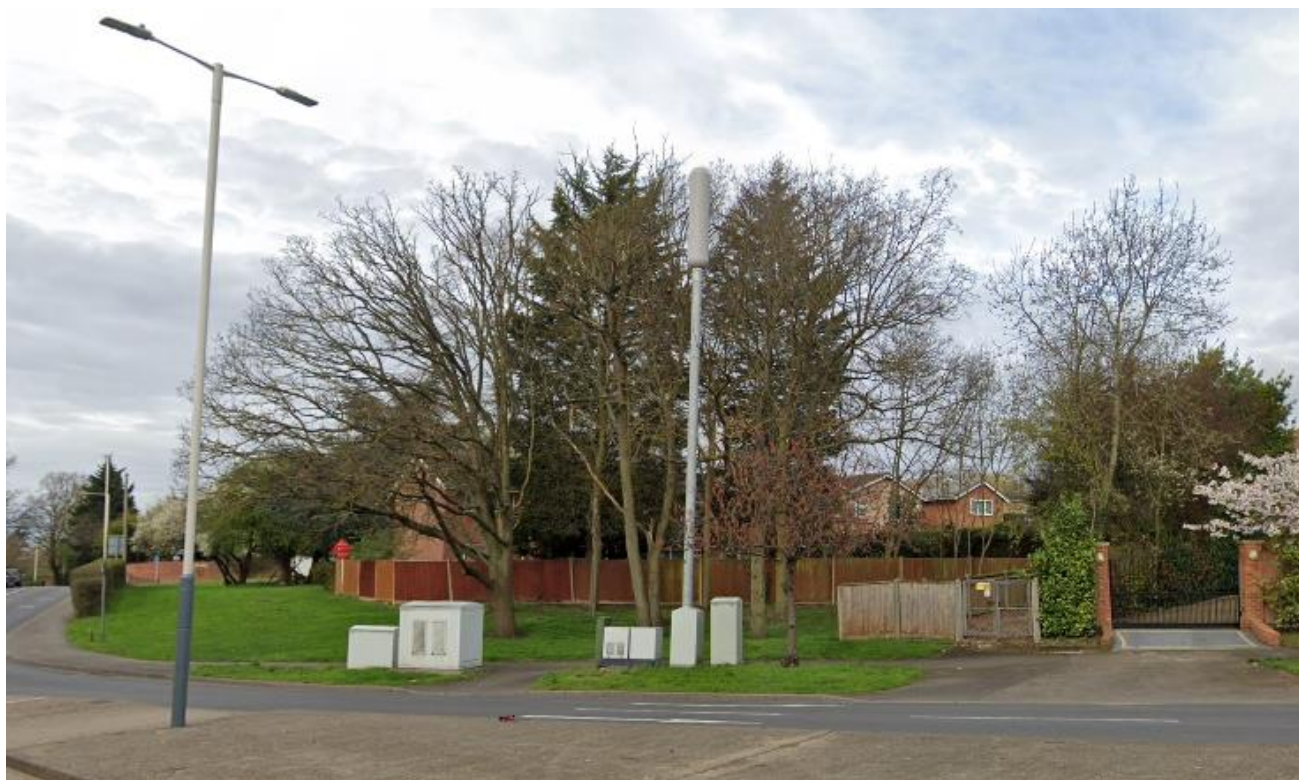
Image 1: Existing MBNL 2G/3G/4G site
