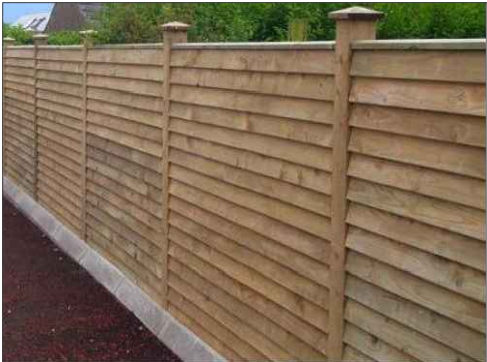
CLOSE BOARDED TIMBER FENCE 1.8M HIGH
