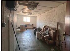
EXISTING STORAGE SPACE ON FIRST FLOOR
