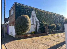
VIEWS TO EXISTING GREEN WALL
