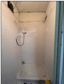
EXISTING SHOWER SPACE ON FIRST FLOOR
