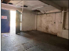
EXISTING OPEN SPACE AND MAIN ENTRANCE INTO THE PROPERTY FROM VILLIER STREET ON GROUND FLOOR
