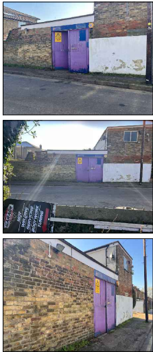
EXISTING VIEWS ALONG VILLIER STREET
