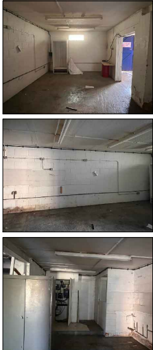
EXISTING STORAGE SPACE ON GROUND FLOOR
