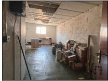
EXISTING STORAGE SPACE ON FIRST FLOOR
