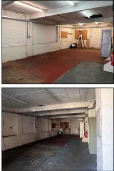
EXISTING OPEN SPACE ON GROUND FLOOR
