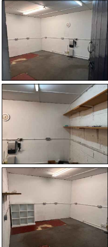
EXISTING OFFICE SPACE ON GROUND FLOOR
