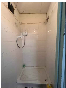
EXISTING SHOWER SPACE ON FIRST FLOOR
