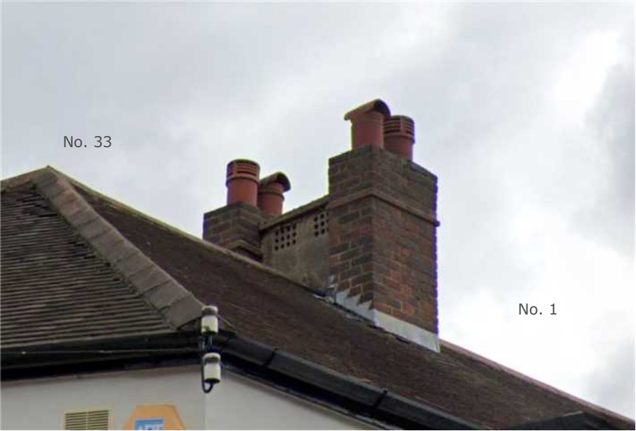
Roof and chimney detail
