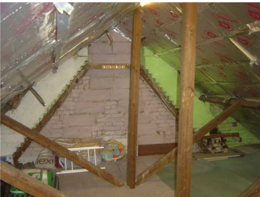
Attic - Chimney breast detail
