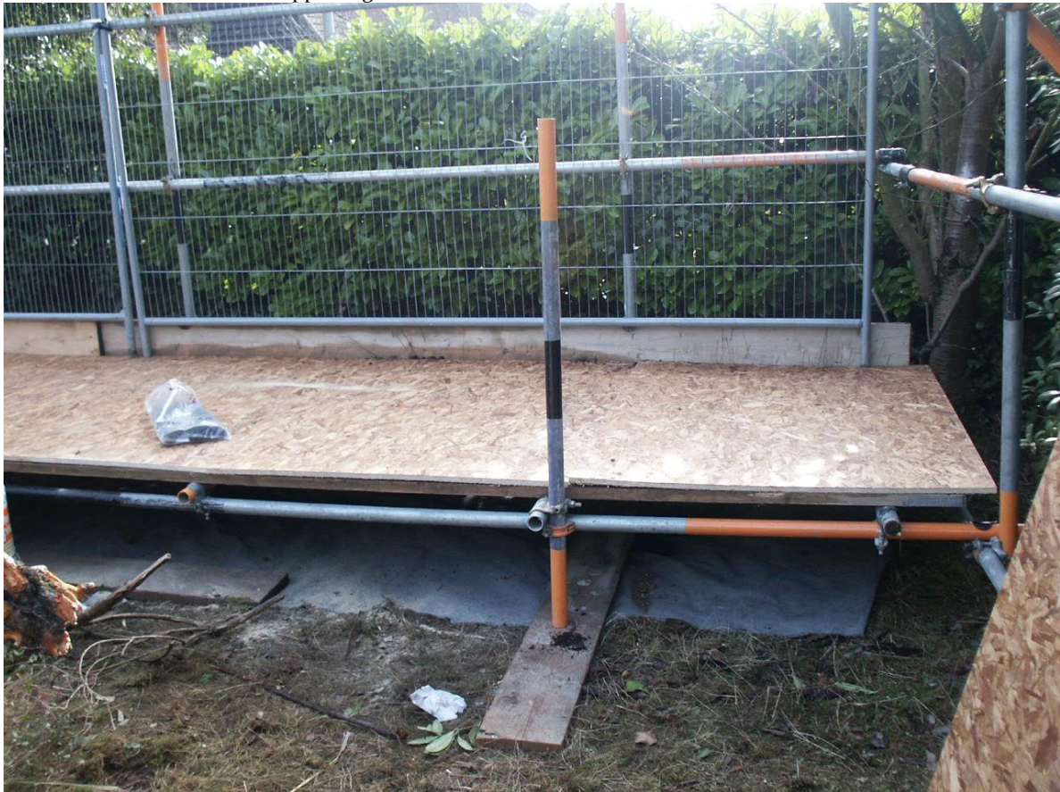
Photo 2 Scaffold framework supporting wooden boards
