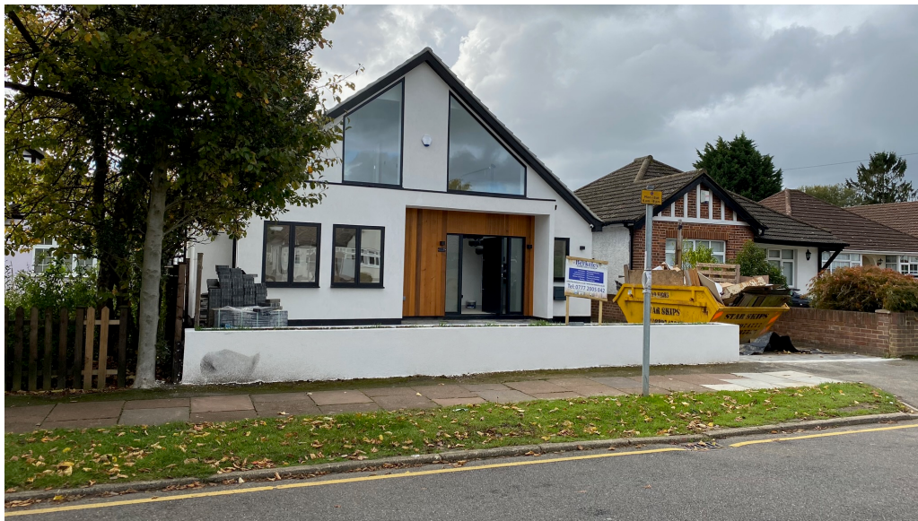
Fig.8 - View of No. 3 Halford Road
