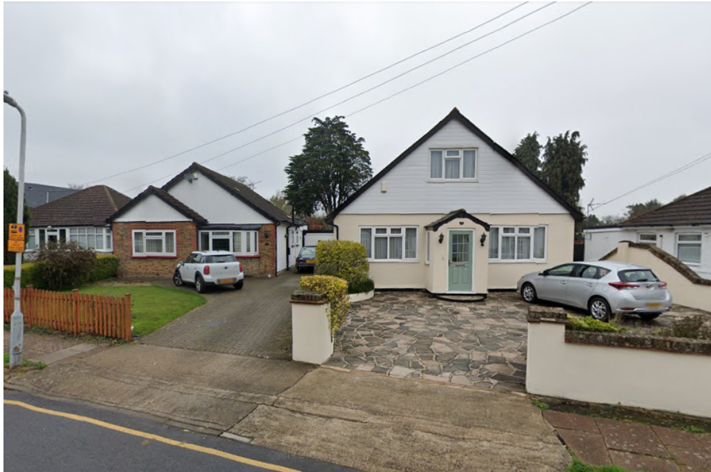
Fig.3 - View of No. 17 & No. 19 The Chase
