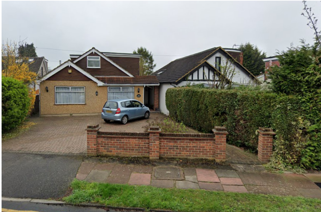
Fig.5 - View of No. 25 & No. 27 The Chase
