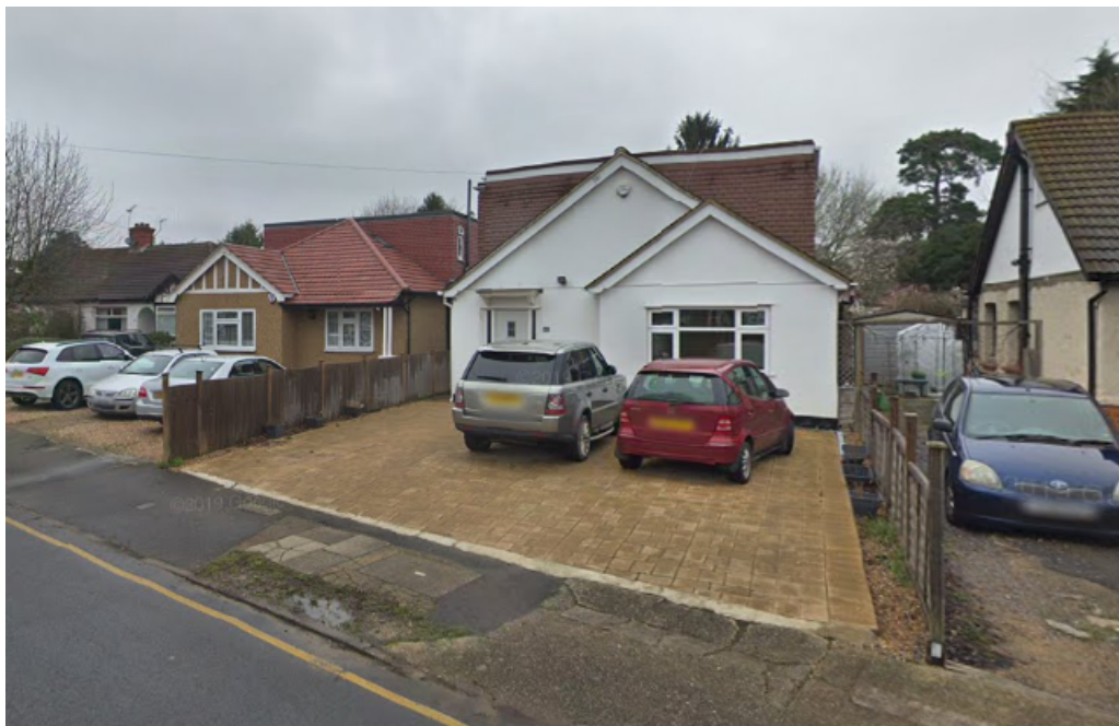
Fig.6 - View of No. 43 & No. 45 The Chase
