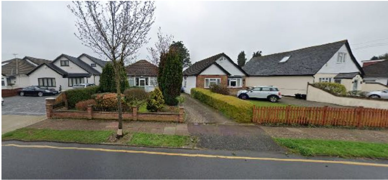
1. View looking North towards front of property No.15 The Chase showing the neighbouring properties and boundaries. Note higher ridges of neighbouring properties.
