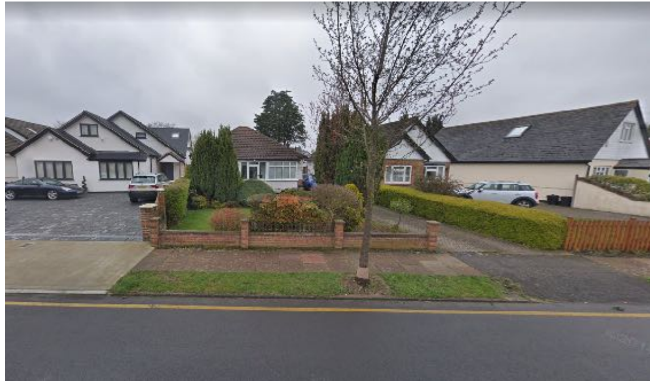
1. View looking North towards front of property No.15 The Chase showing the neighbouring properties and boundaries. Note higher ridges of neighbouring properties.
