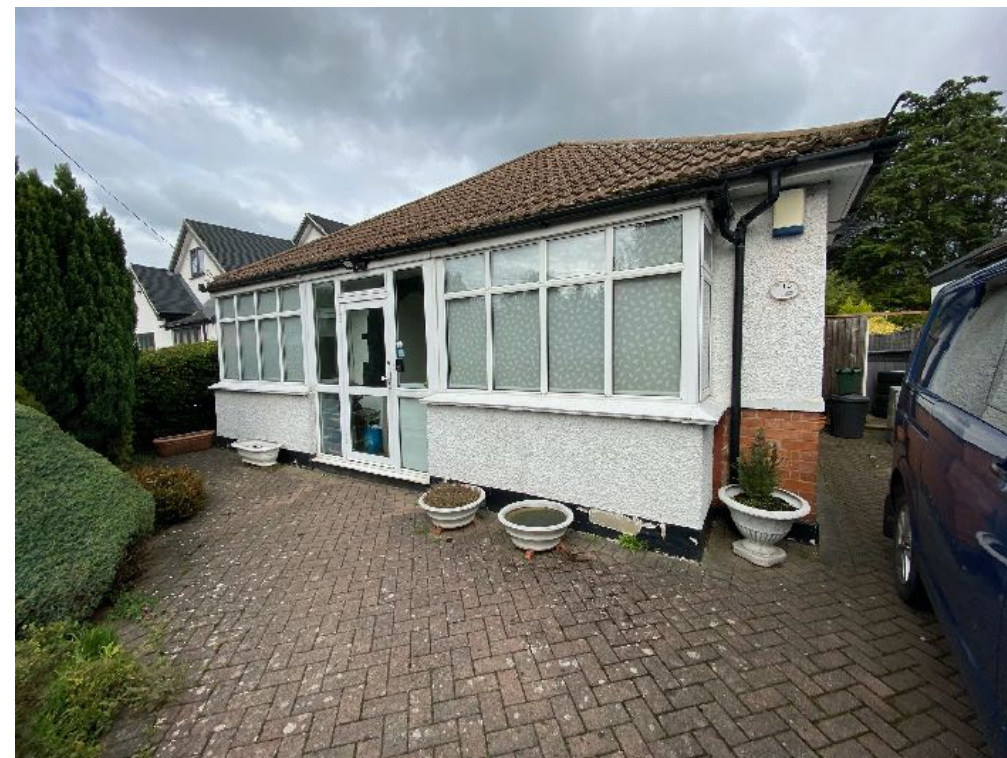
4. View looking North-West towards the front of property No.15 The Chase showing existing infill porch.
