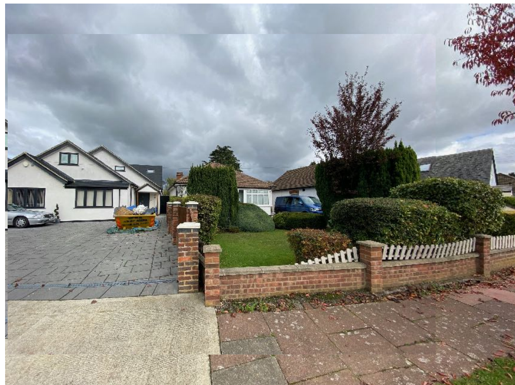
3. View looking North towards front of property No.15 The Chase showing the neighbouring property and boundary No.13 The Chase. Note higher ridge and gable end design, similar to thst of the application scheme.
