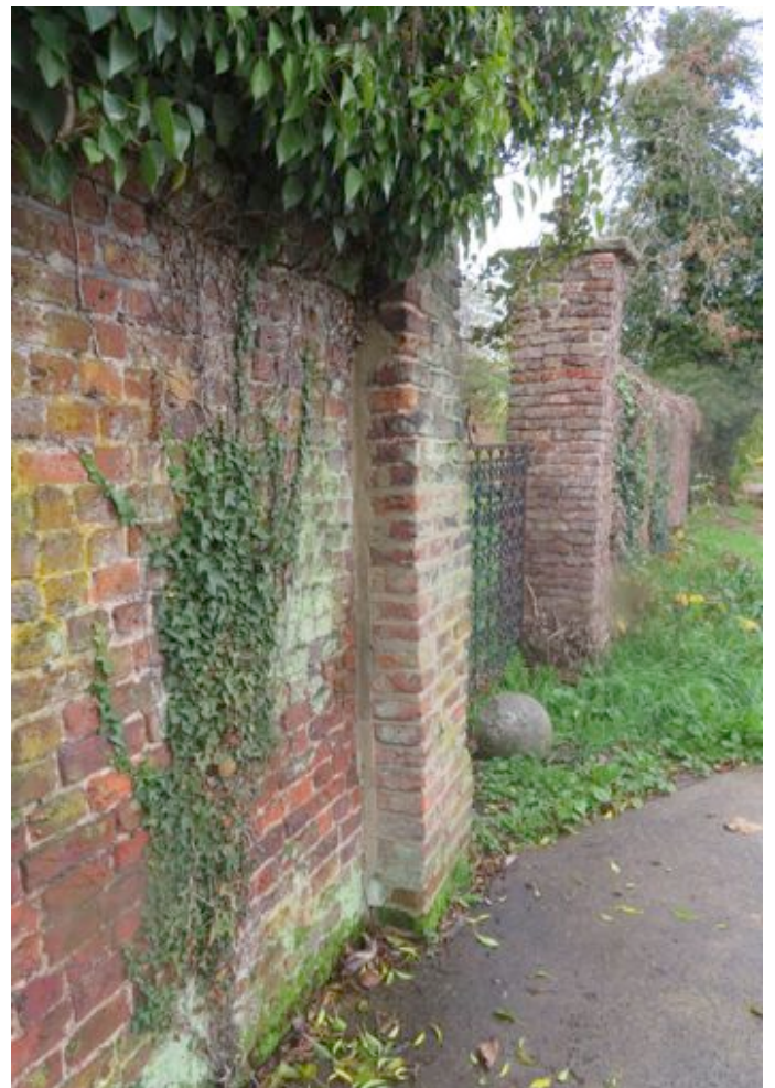
East face of pier looking north
