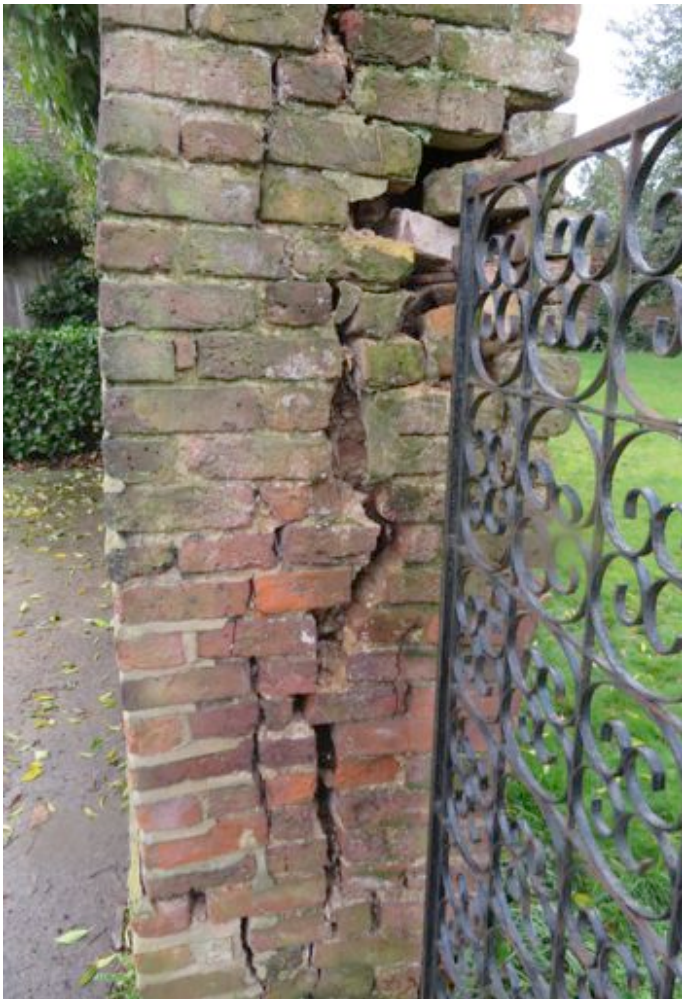
North face of pier
