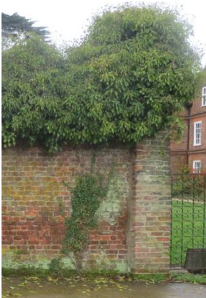
East face of pier, looking west
