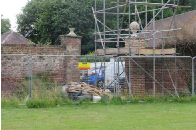
General view on completion. West side.
