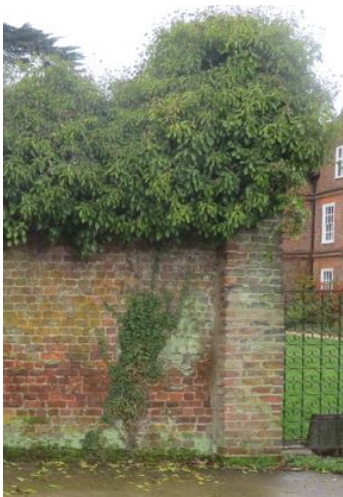
East face of pier, looking west
