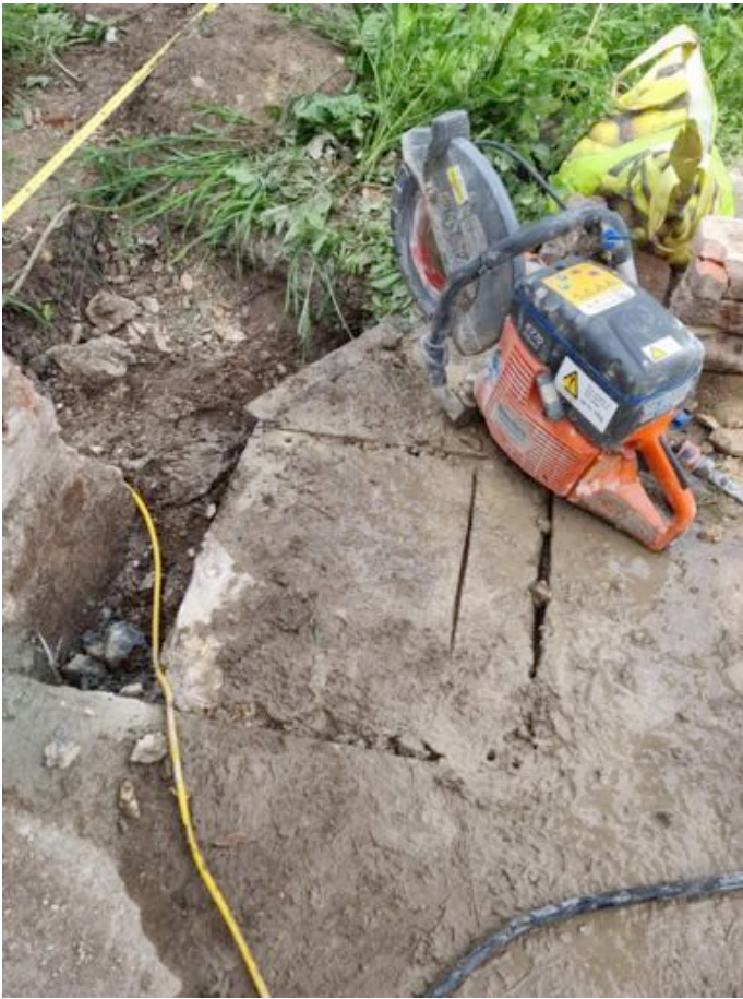
Cutting away concrete at the base of the east side of the pier.
