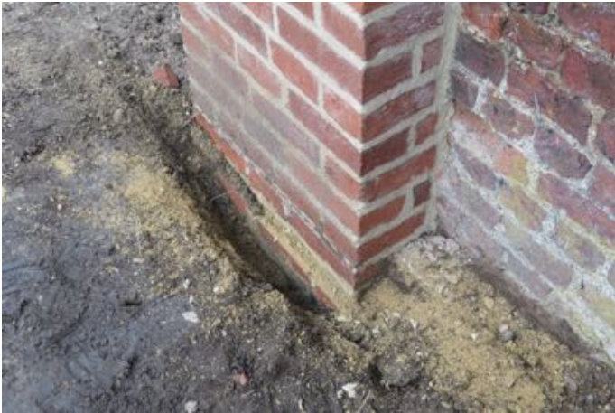
Ground part re-excavated to show foundation on west side
