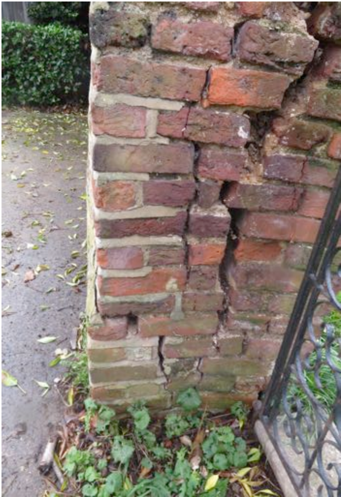
North face of pier
