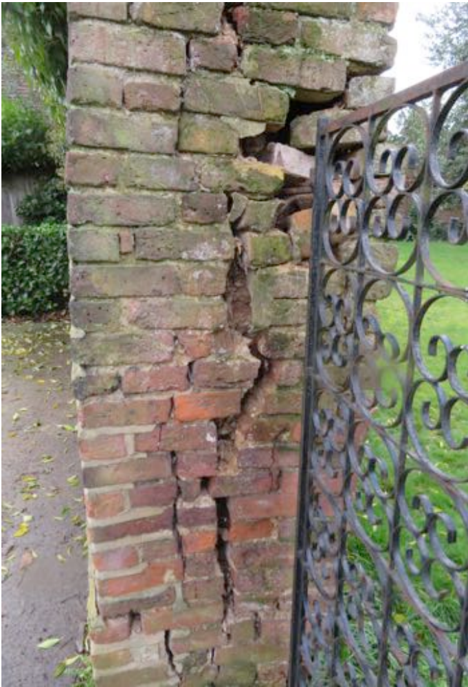
North face of pier
