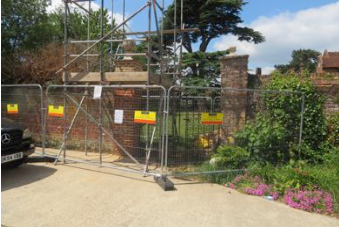
General view on completion. East side.
