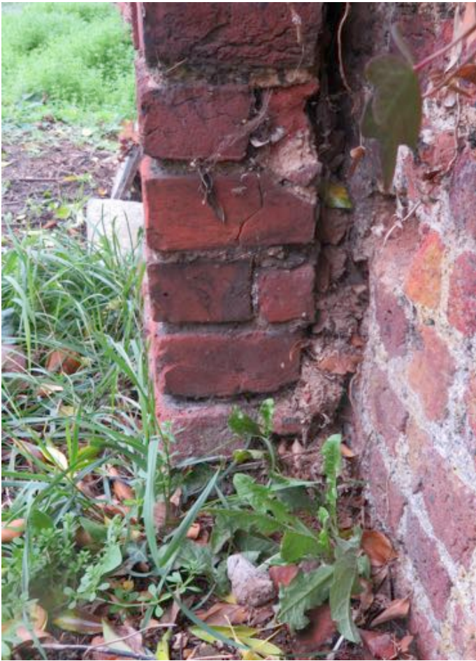
Base of west face of pier, looking north.
