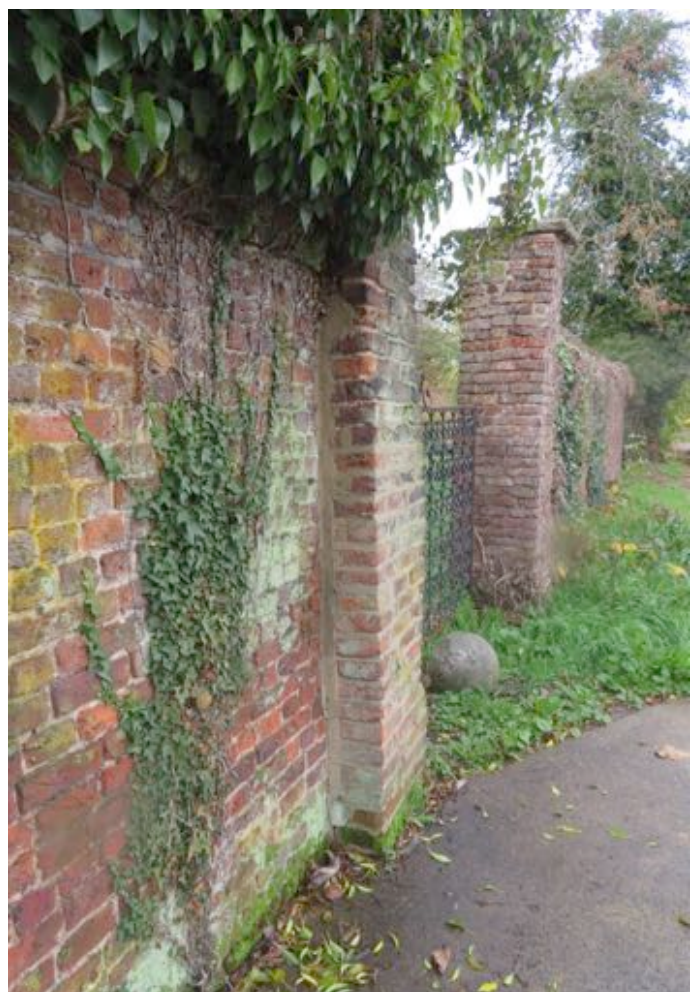
East face of pier looking north
