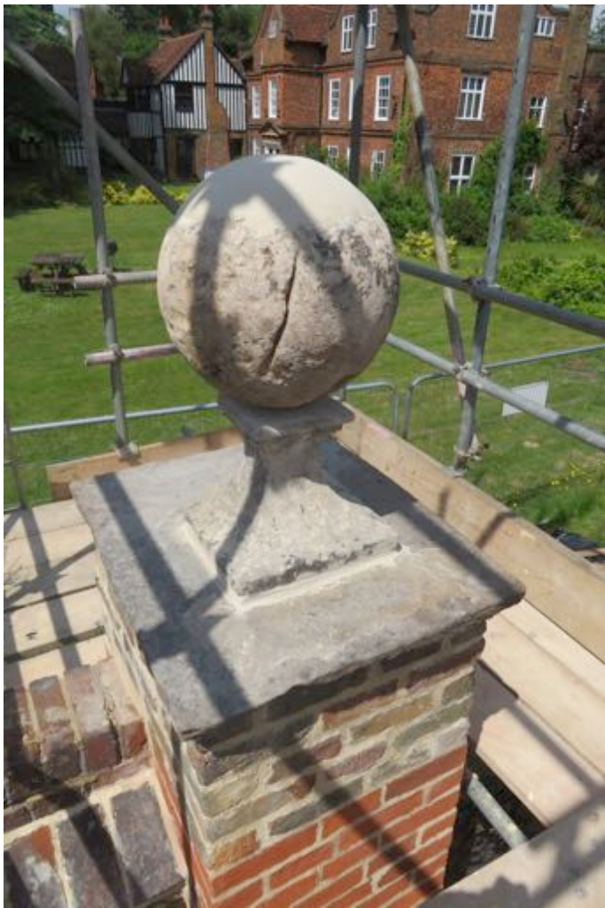
Pier cap on completion. East side.
