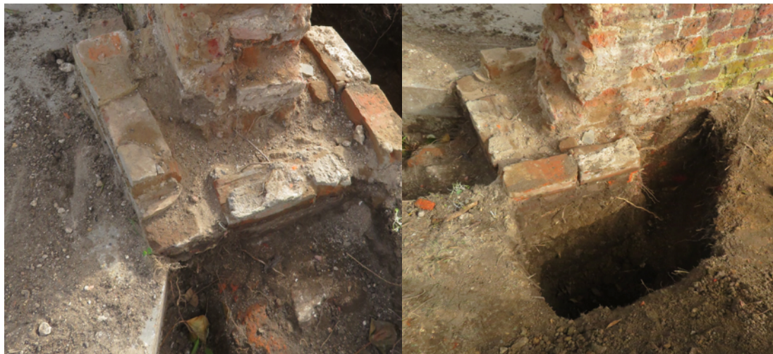
Base of the pier viewed from the NE. The original foundation to the historic wall can be seen at the base of the photo and the thick concrete slab to the left.
