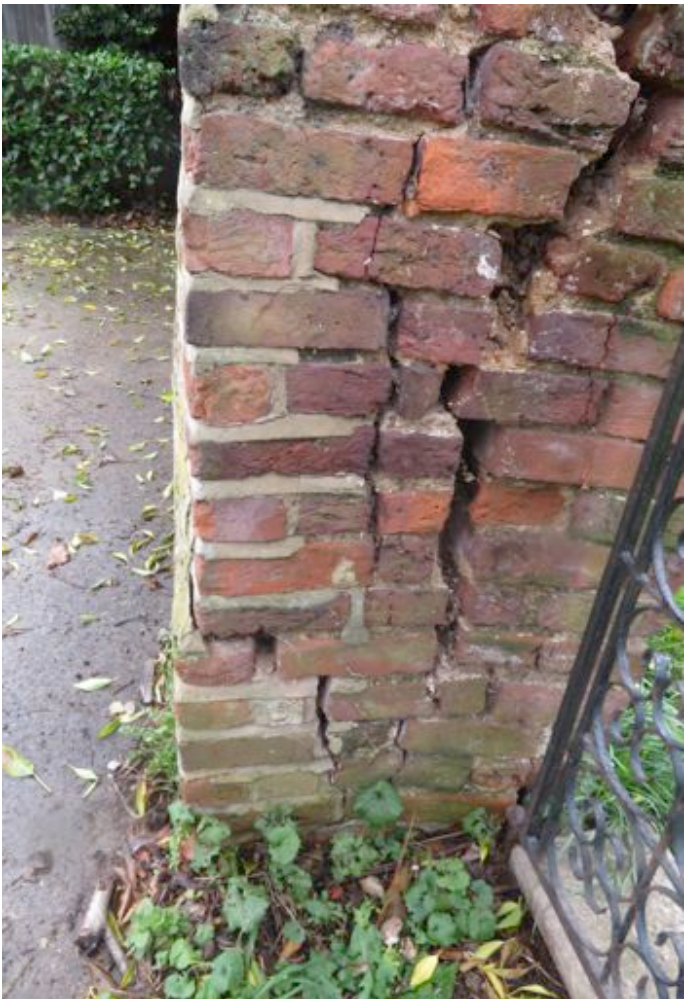
North face of pier
