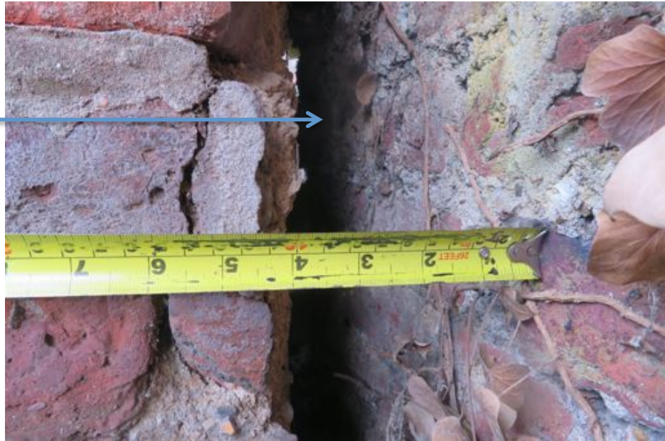
WEST FACE OF THE PIER
