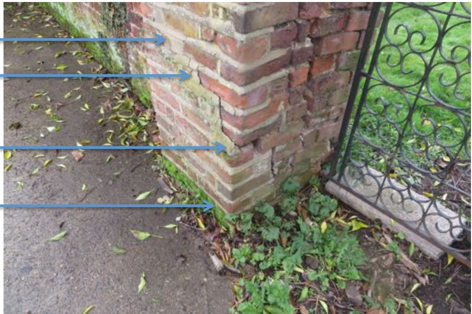
NE CORNER OF THE PIER.
