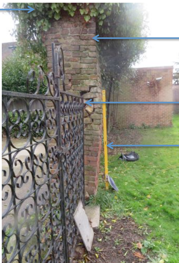
NORTH FACE OF THE PIER
