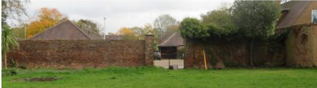
View of the west side of the wall
