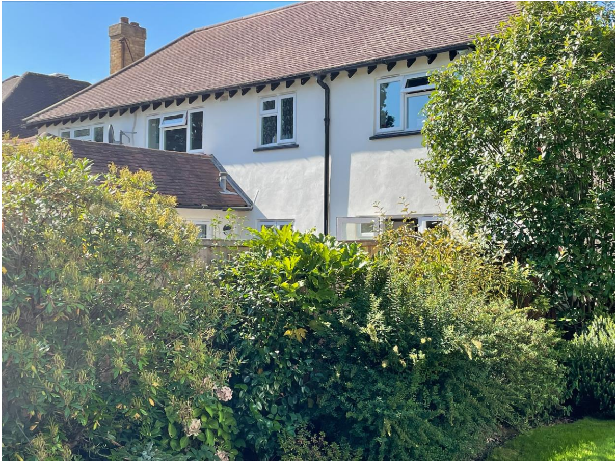
Agent Site Photos – 19 Highfield Drive Ickenham Received 24/09/2021
