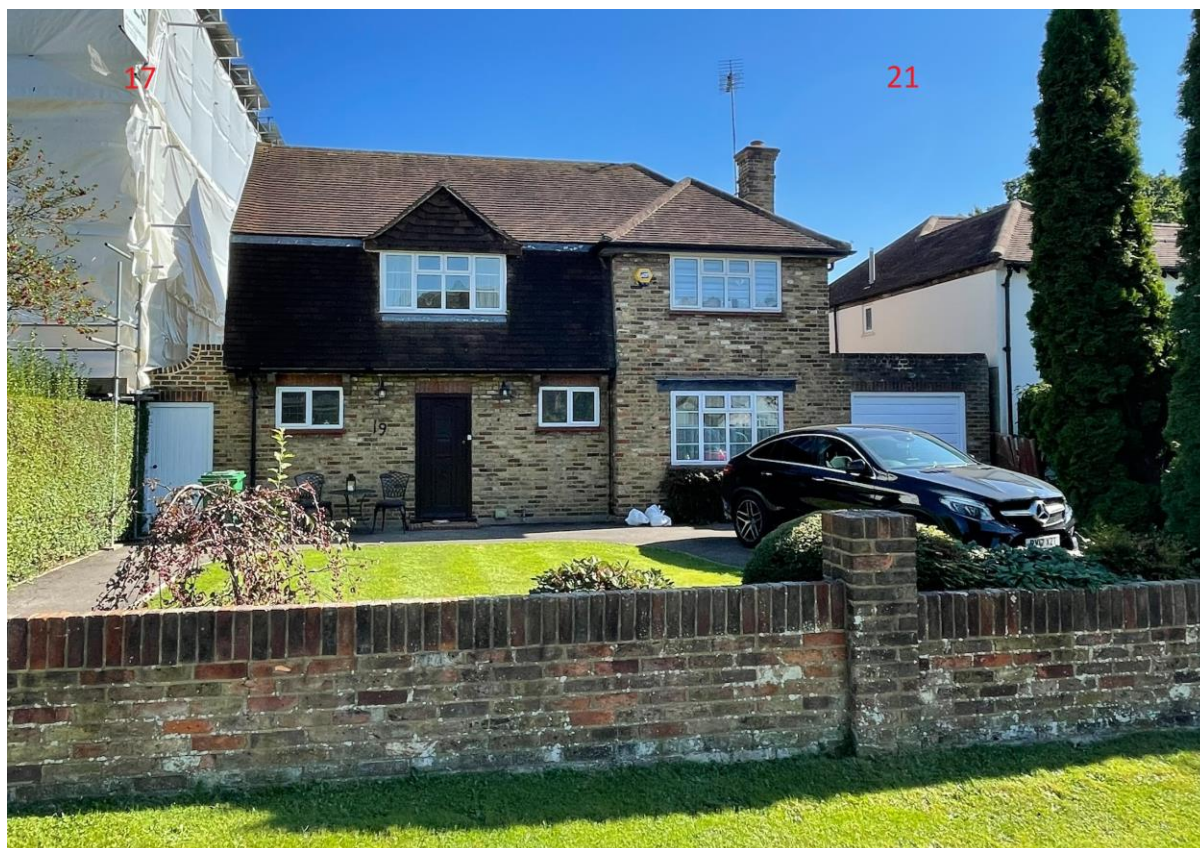
Agent Site Photos – 19 Highfield Drive Ickenham Received 24/09/2021
