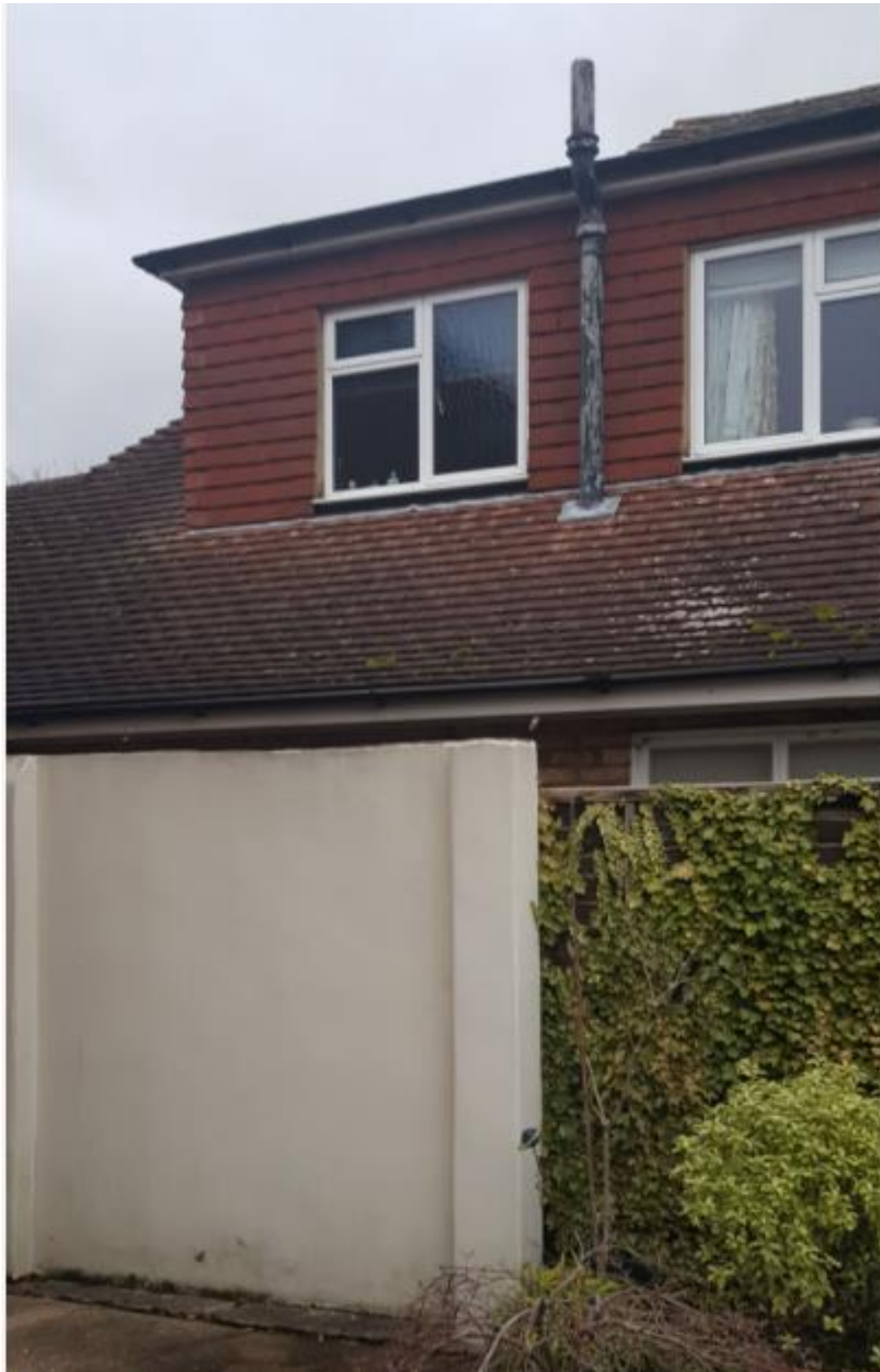
Agent Site Photos – 19 Highfield Drive Received 03/12/2021 – Side/Rear of no.17
