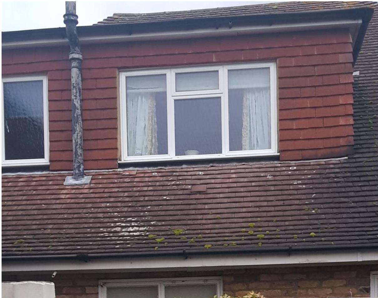
Agent Site Photos – 19 Highfield Drive Received 03/12/2021 – Side/Rear of no.17
