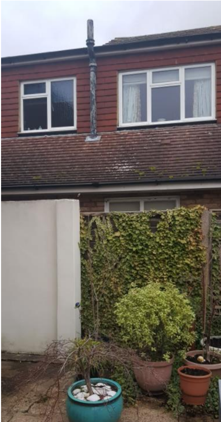
Agent Site Photos – 19 Highfield Drive Received 03/12/2021 – Side/Rear of no.17
