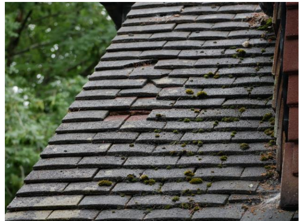
Plate 3.6: Slipped Tiles
