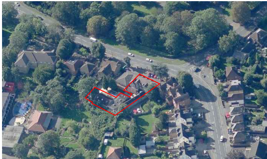
4 Aerial View View from the North
