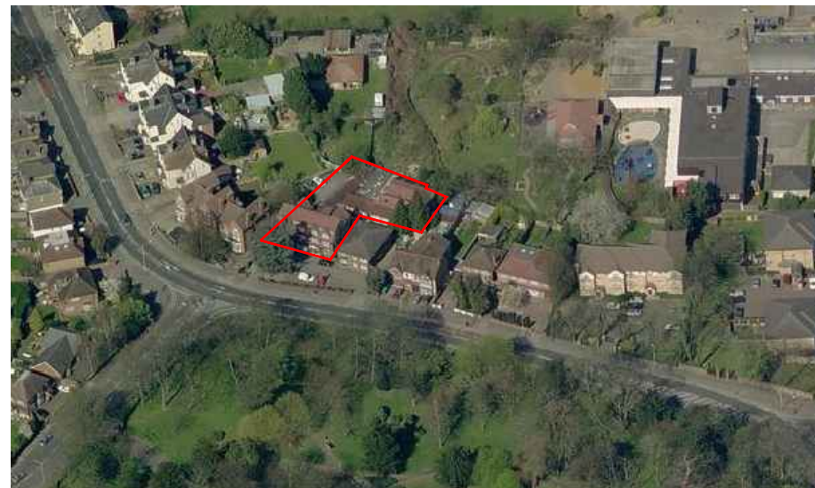
3 Aerial View View from the South
