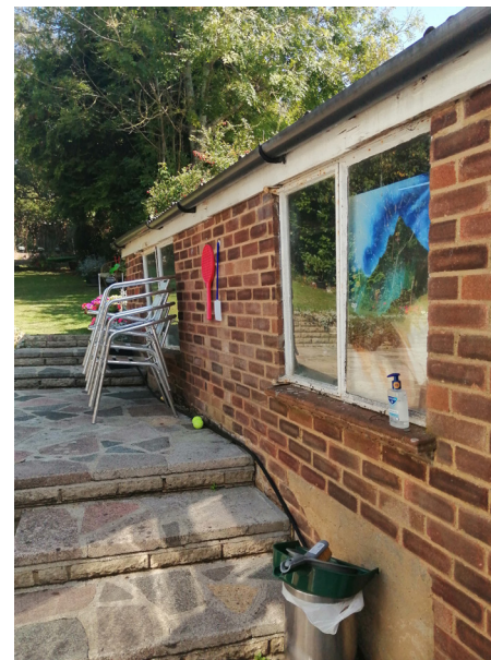
Garage of No.85 Hillside Road
