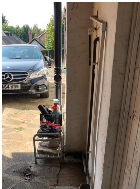
Side of No.85 Hillside Road
