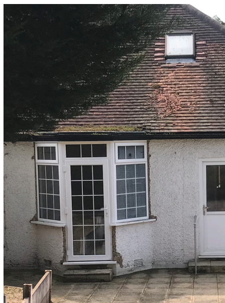
Rear of No.83 Hillside Road
