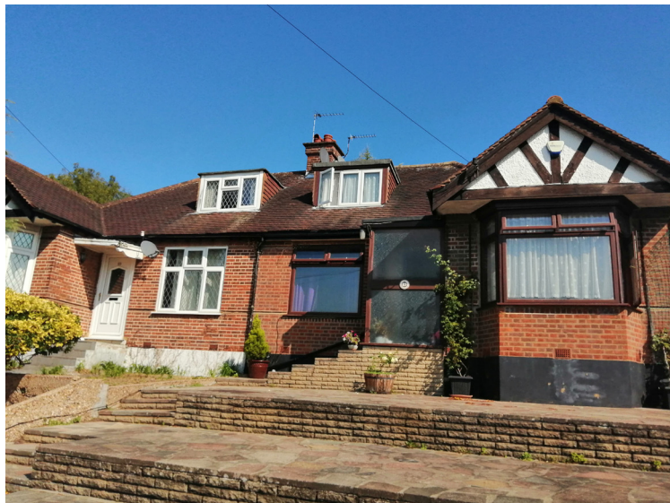
Front of No.83 & 85 Hillside Road
