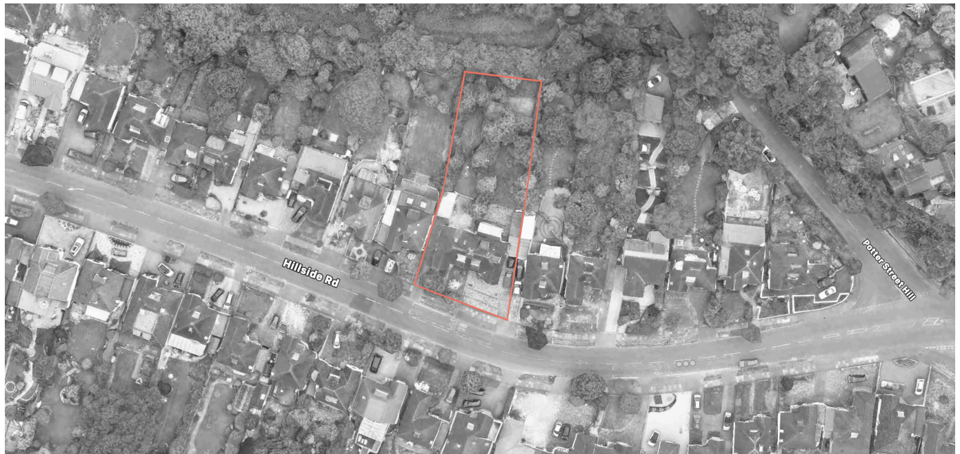
Aerial view with the subject site in red boundary (not to scale)
