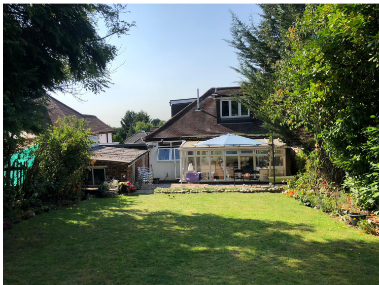
Rear of No 85 Hillside Road
