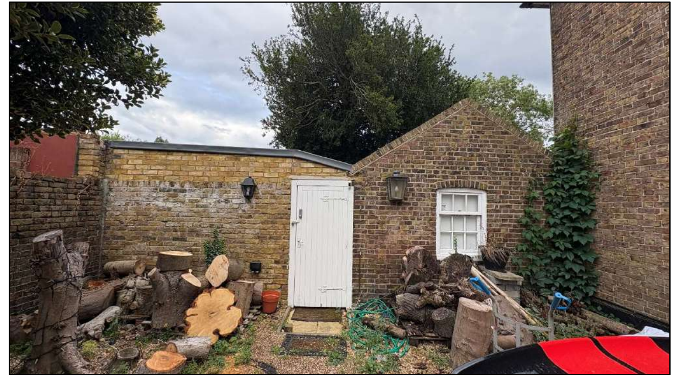
Image 20: Roof Closure to Courtyard
