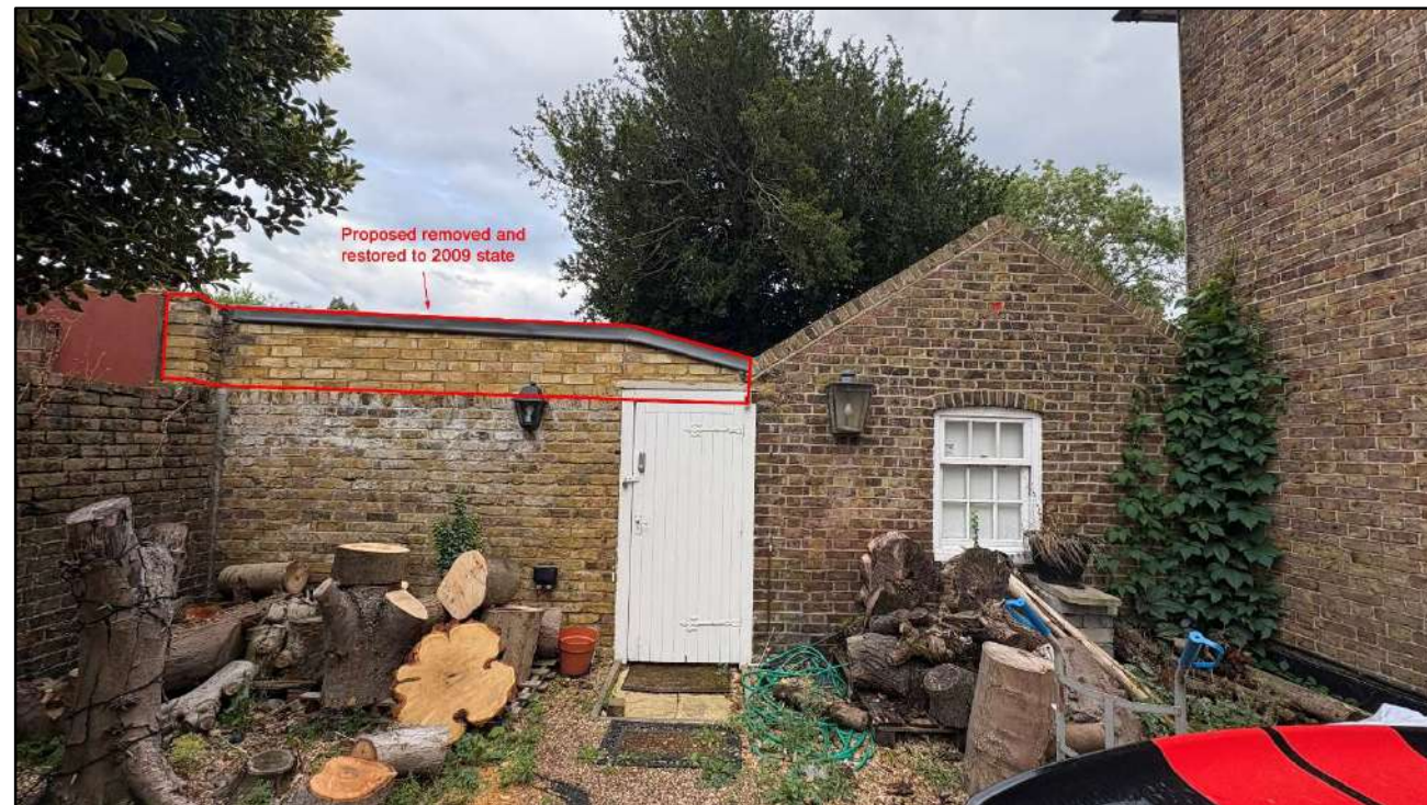
Image 43: Removal of Roof Closure to Courtyard and Additional Brickwork
