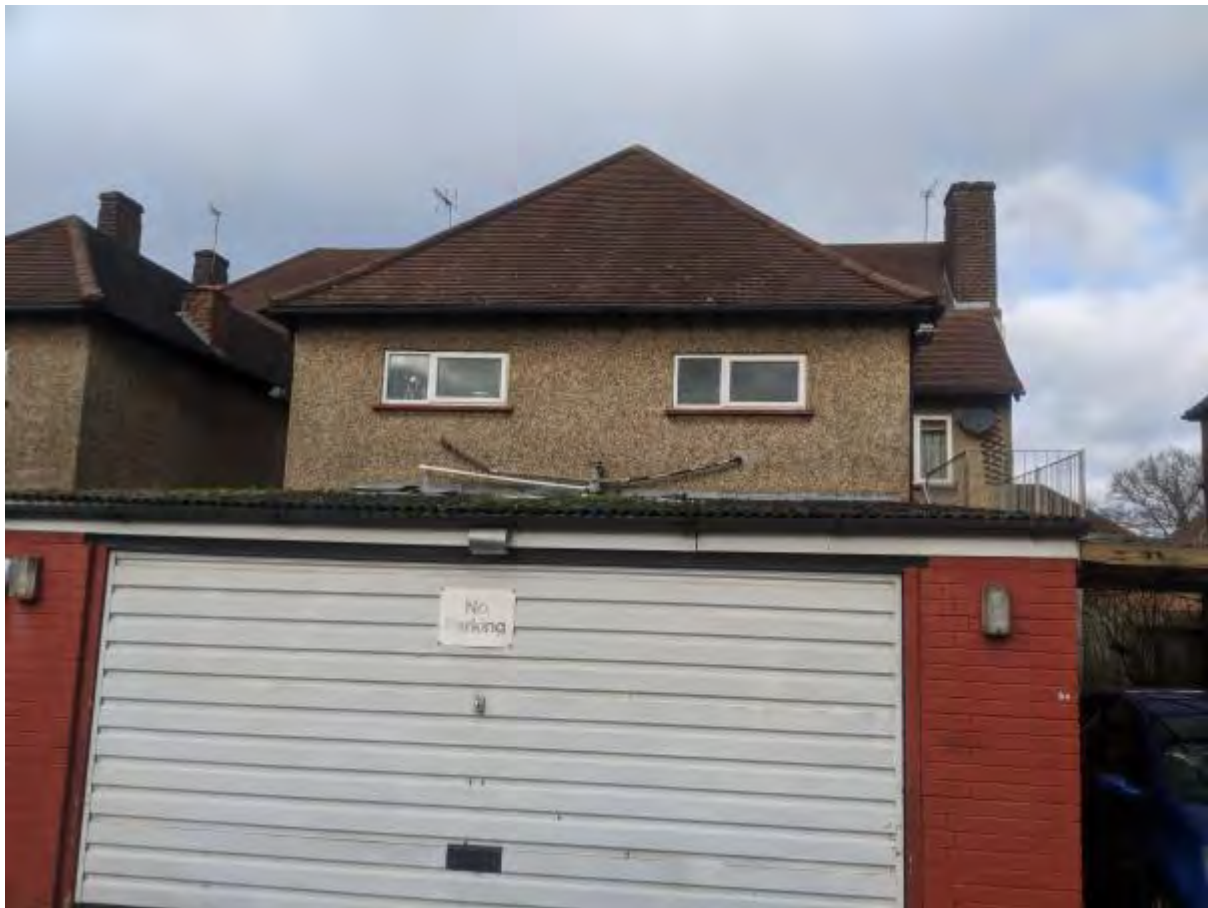
PLATE 2: Garage with possible asbestos roof
