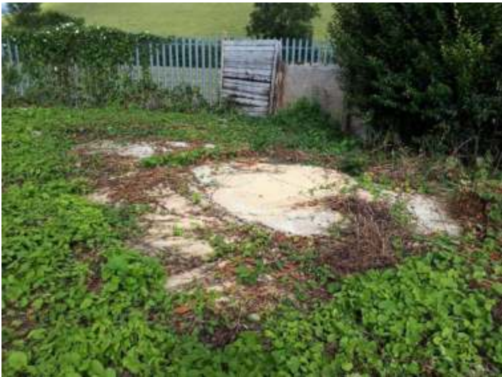
Plate 12: Hardstanding (concrete) on site, approximately 7 m x 3 m in size.
