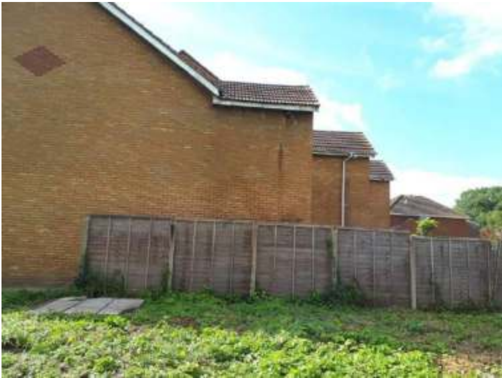
Plate 7: Viewing south from the site – 73 Stanwell New Road.
