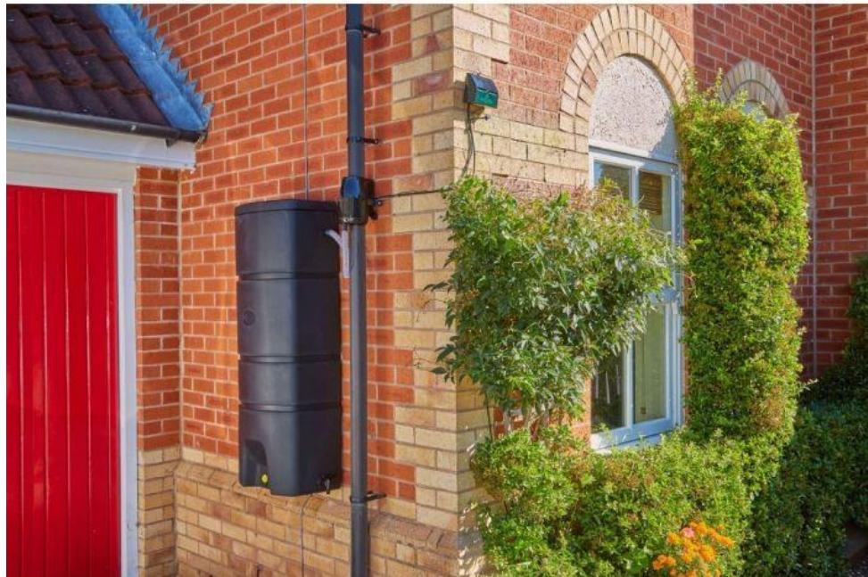
The slimline rainwater harvesting/water butts for external use will provide additional, "off line" SuDS, and is a suitable SuDS component for small plots. The collection and re-use of water will reduce run off volumes arising from roofs. The collected water, via diverters will be used for external uses with manual control. Any useful volume is not accounted for in storage calculations
