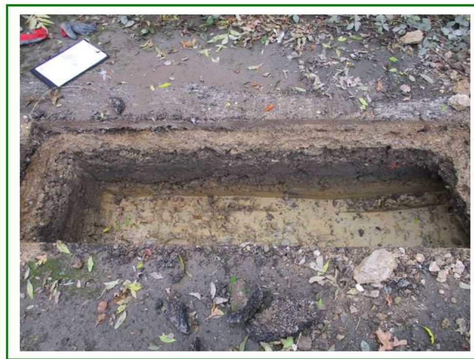
Photo No.2: TP01 pit sides and base (excavated through tarmac and concrete base)
