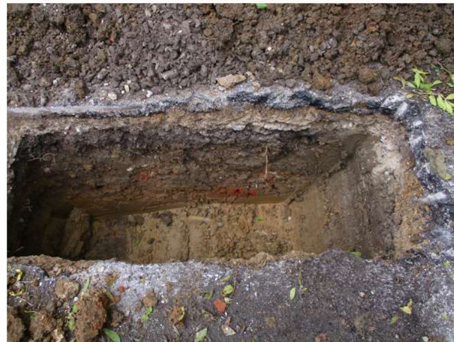
Photo No.6: TP03 pit sides and base (excavated through tarmac and concrete base)
