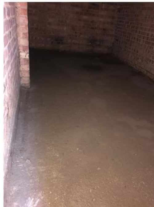
Photo No.4: Facing south west showing interior of a garage unit showing concrete flooring and no staining or damage
