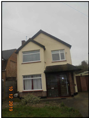
Existing Front View
