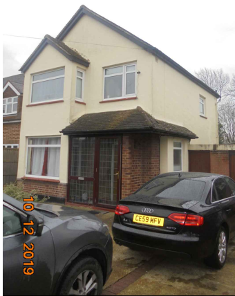
Existing Front Corner View
