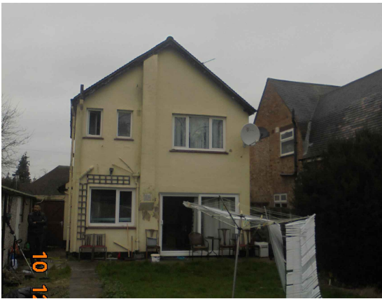
Existing Rear View
