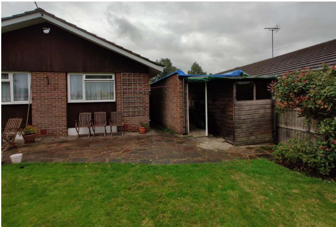
Rear of garage
