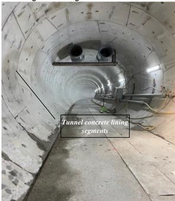
Figure 7: Tunnel Segmental Lining
