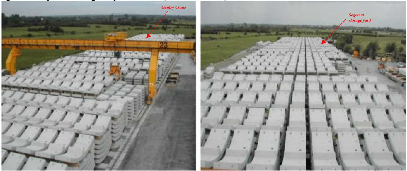
Figure 8: Gantry crane and segment yard illustrated (Dublin Port Tunnel)
