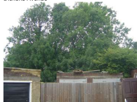
Views at end of garages towards rear two garages (see plan)
