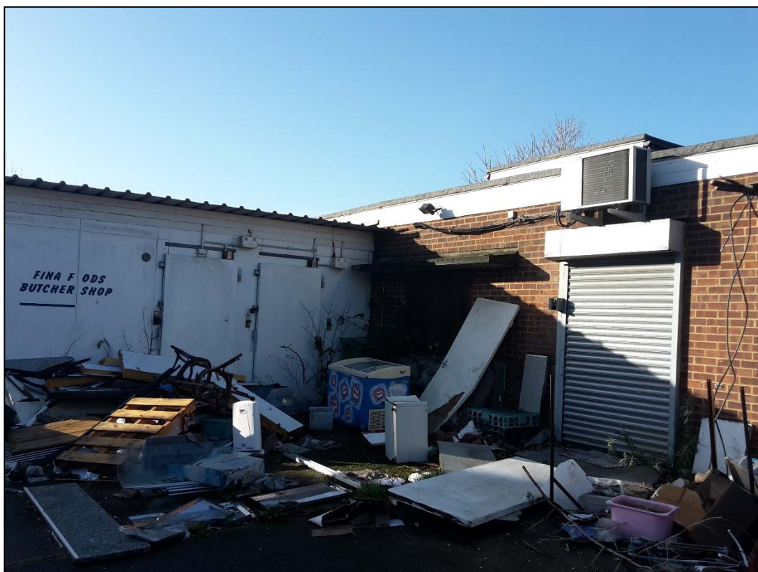
Photograph 3 – Evidence of fly tipping and former commercial use of buildings on site.
