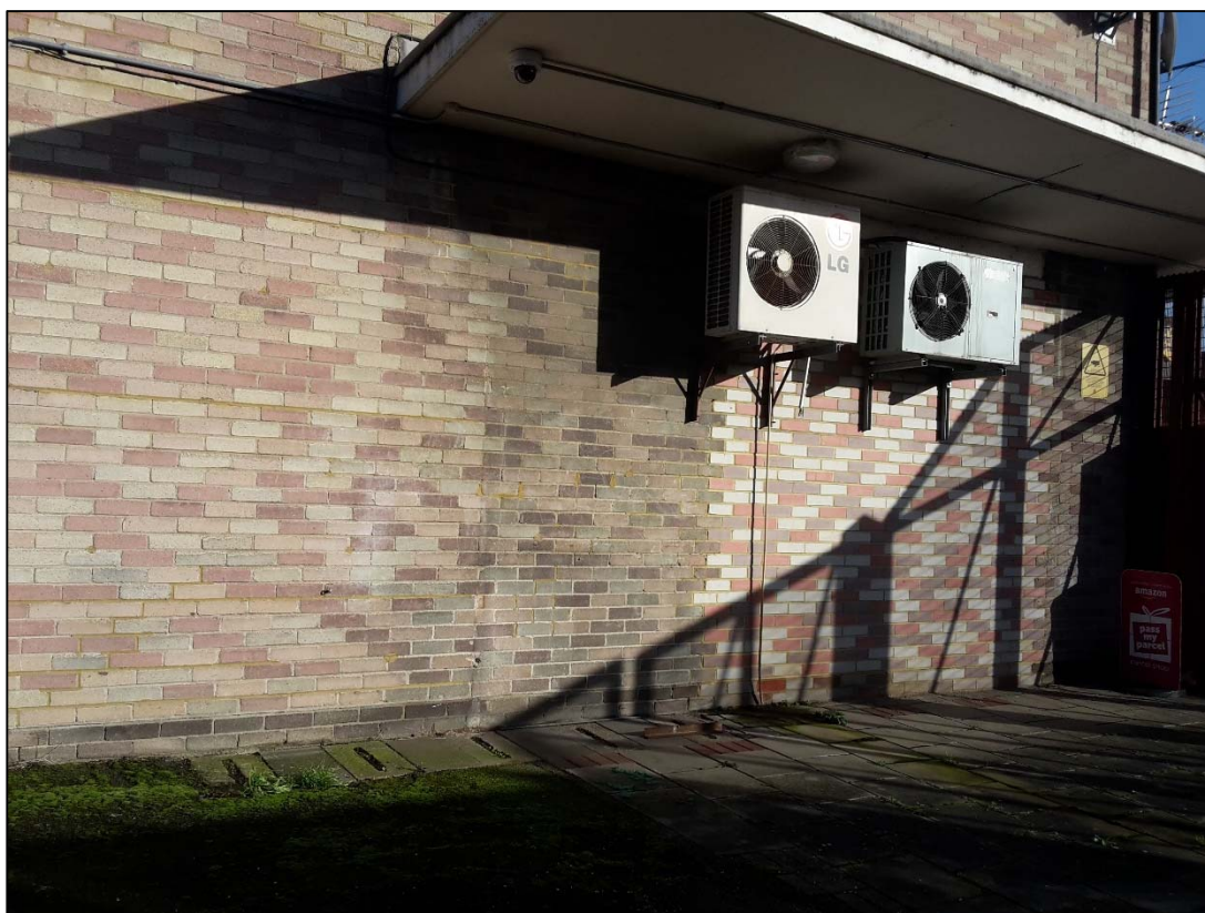
Photograph 5 – Air conditioning units and altered brickwork immediately to the south east of the site.
