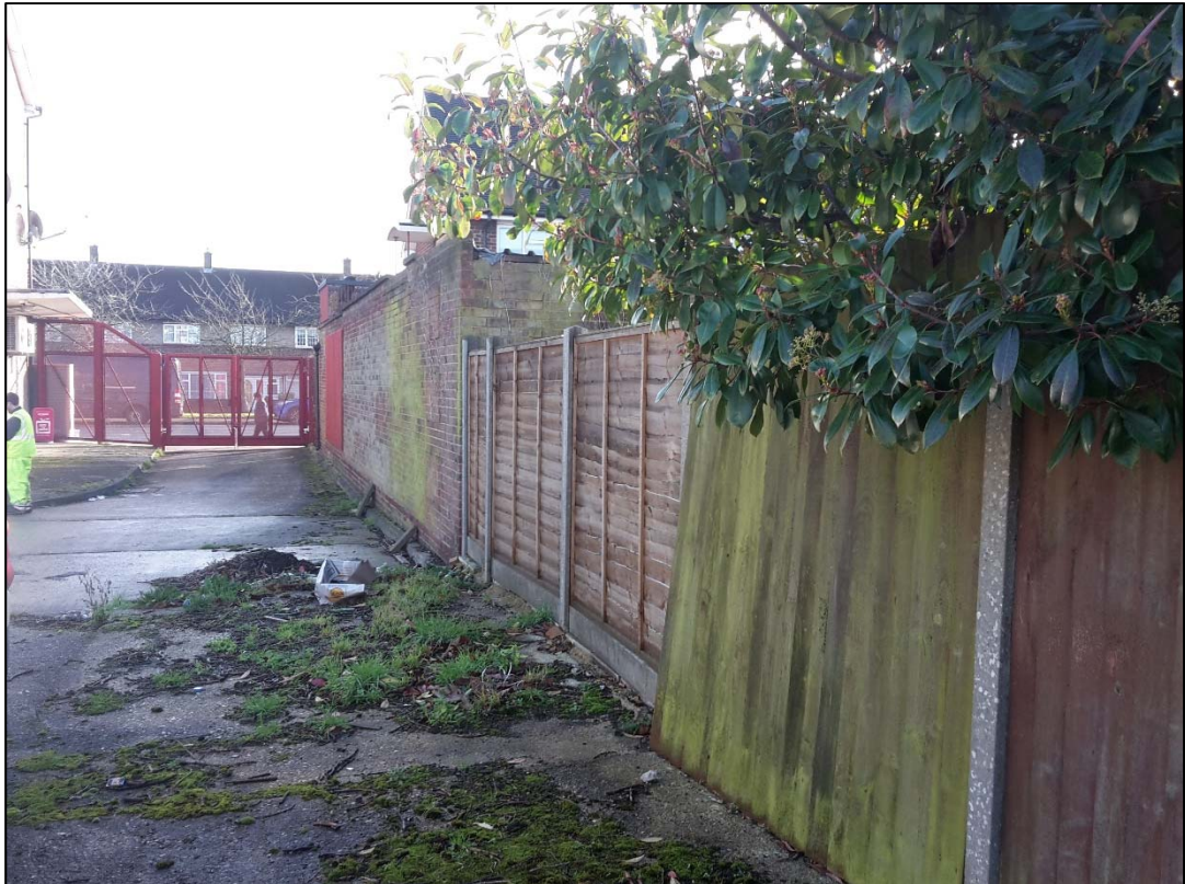
Photograph 1 – Looking east along the southern site boundary.
