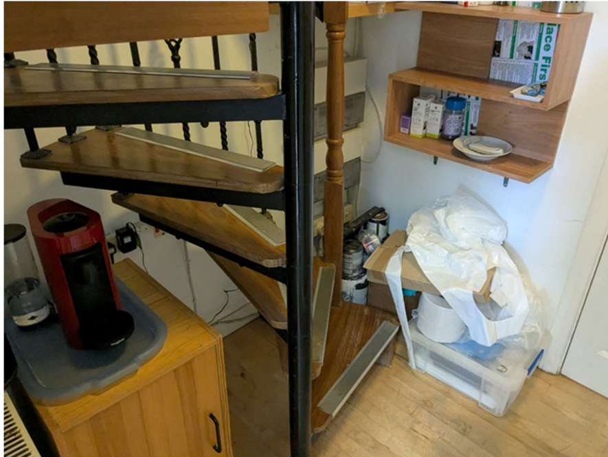
The current spiral circulation staircase is wholly unsuitable
