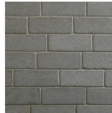
Brick (Plinth & Bay window)
