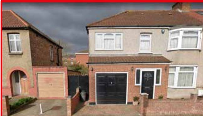
There is a 1.6 metre gap at ground floor and 3.8 metres at first floor.
