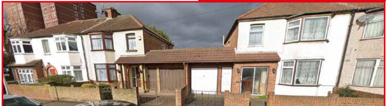
Single storey extensions abutting with no gap at ground floor and a 6.3 m gap at first floor. End dwelling is larger than standard but retains the bay window design feature.
