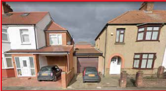
There is no gap at ground floor and 4 metres at first floor.
