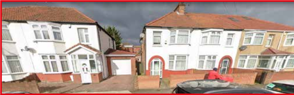
Single storey extension with a footpath gap at ground floor and a 4.65 metre gap at first floor between the terrace and semi-detached properties.
