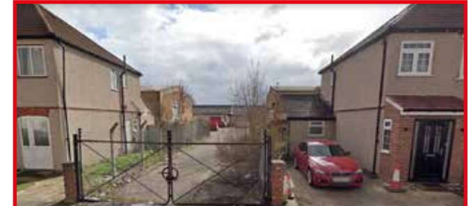
The gap here is a total of 12.759 metres at present and would result in a 2.8 metre gap to the left and 3.8 at first floor with 1 metre gap at ground floor to the right following development.
