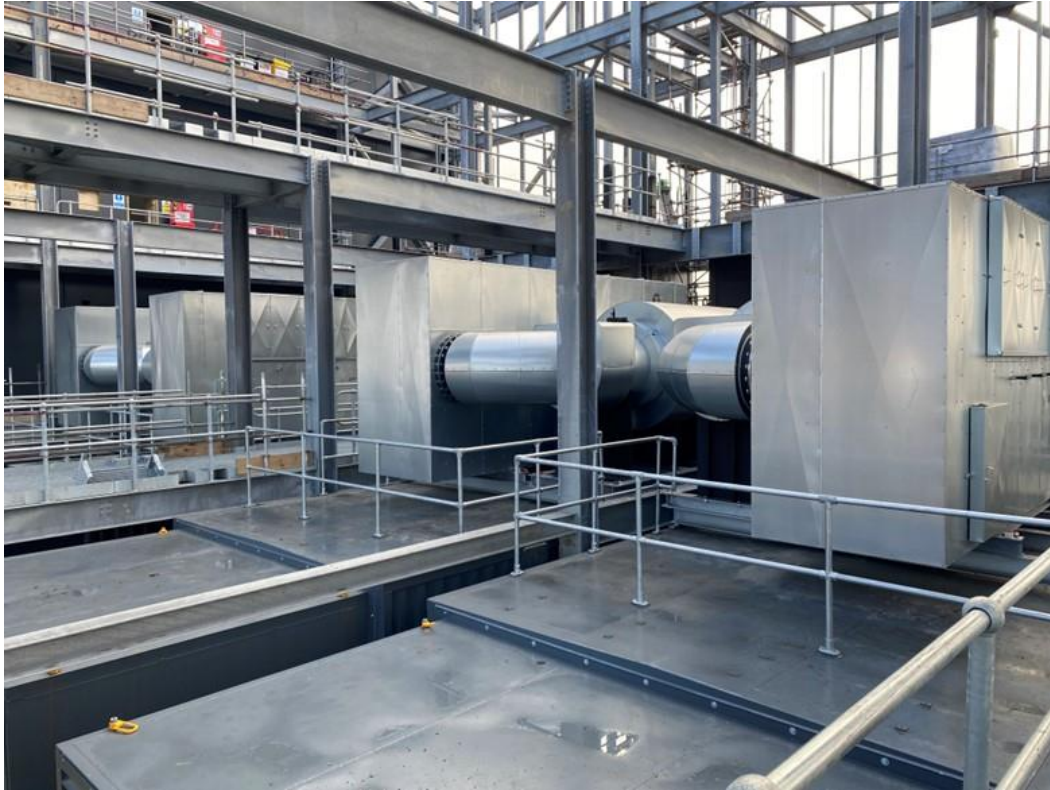
Figure 1 SCR system on top of generator container
