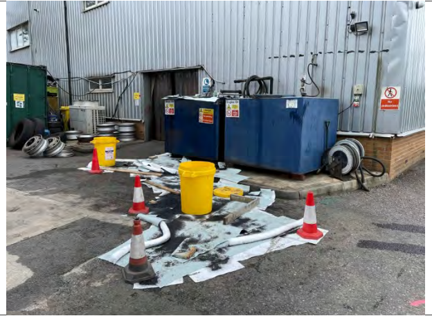
06: ASTs and spill identified at the rear of the building
