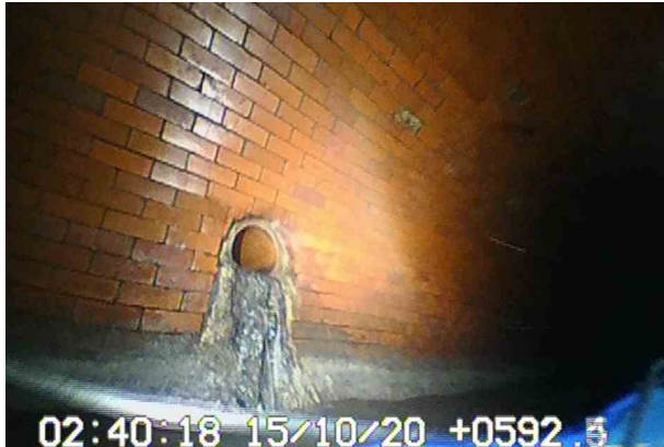
17, 592.80 m Connection other than junction at 9 o'clock, diameter: 225mm, RUNNING
