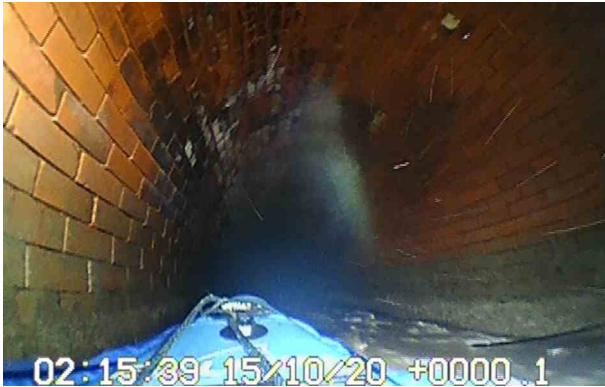
1, 0.01 m General remark, FLOAT SURVEY
