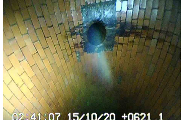
18, 621.30 m Connection other than junction at 12 o'clock, diameter: 300mm, LAMPHOLE
