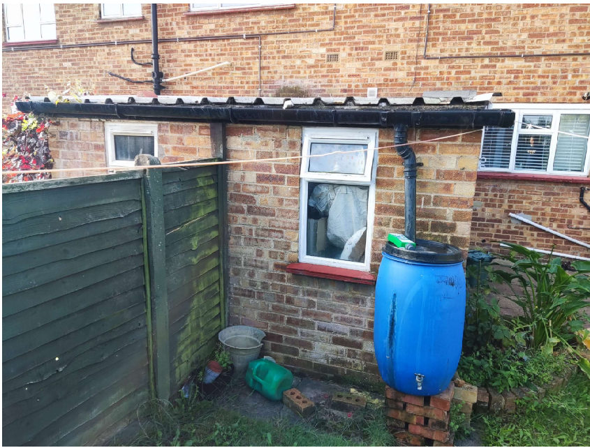
View to the shed
