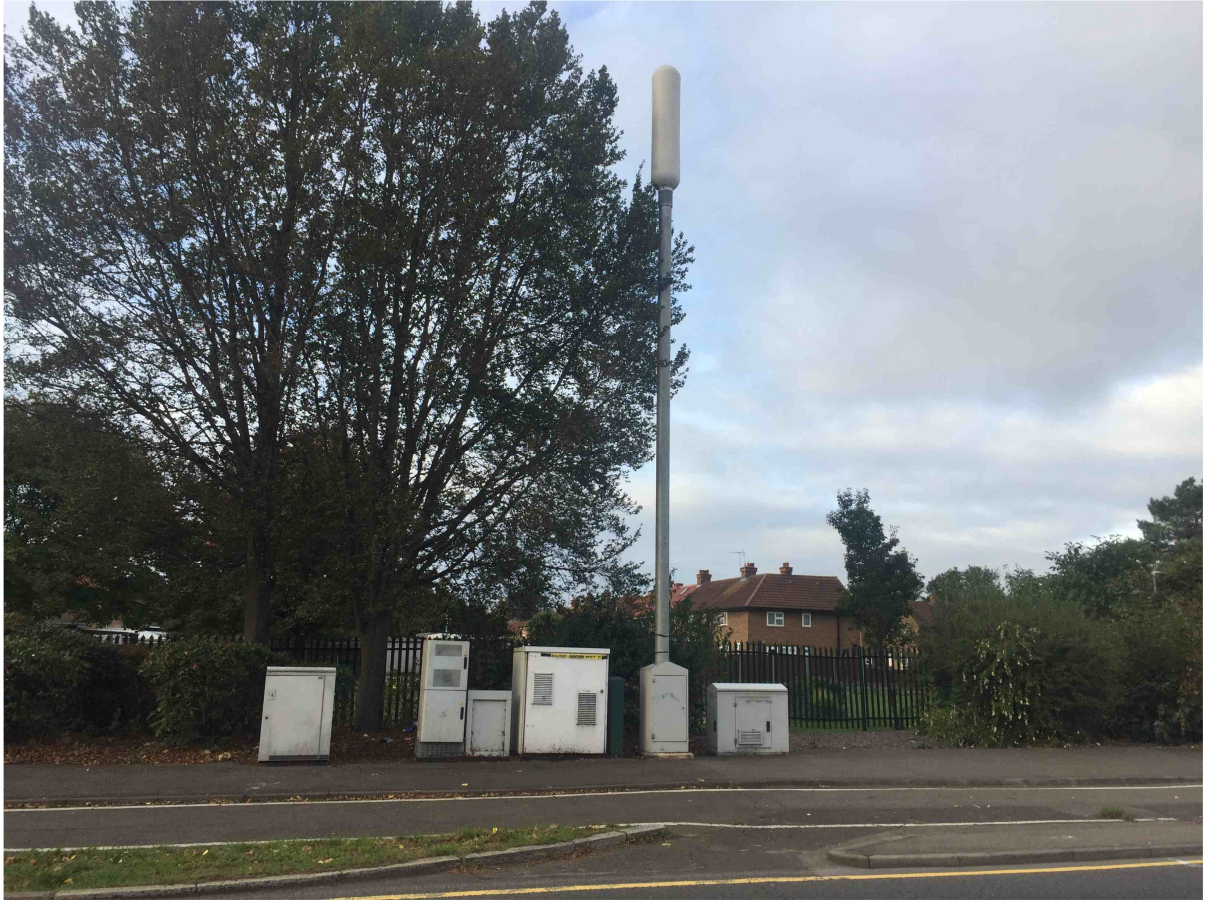
View of existing mast from the South, along Uxbridge Road.
