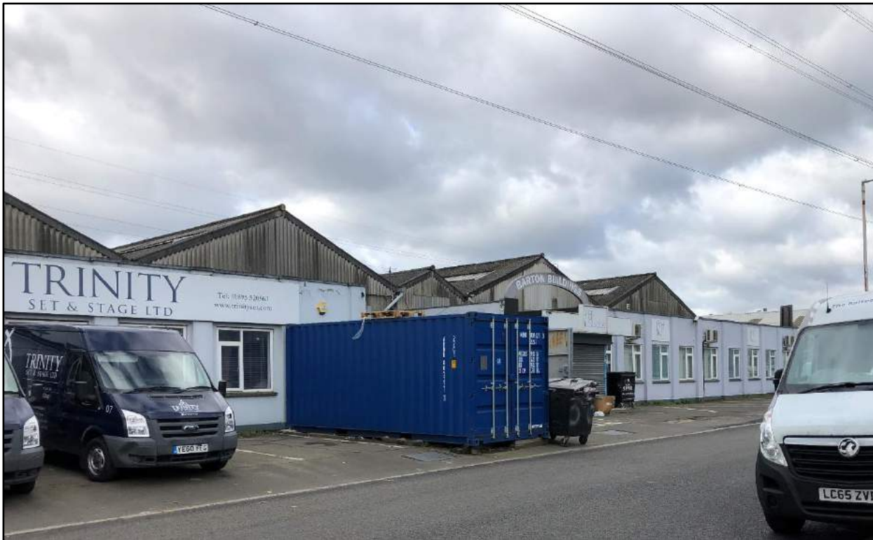
Photograph 1: View of the site from Arundel Road
