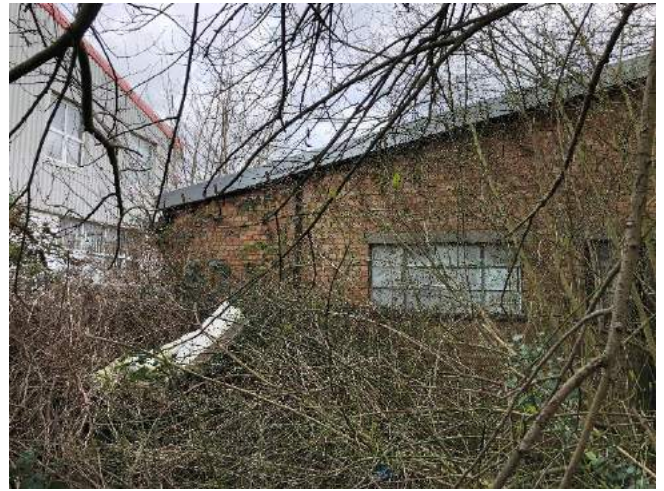
Rear of storage building, view from outside of eastern end of site.
