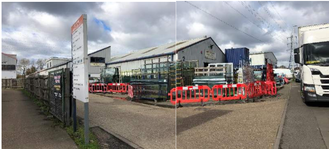
Arundel Road Frontage, Access Road, North Boundary & adjacent site to the North
