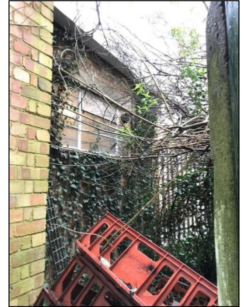
Appendix B Figure 40: View of potential access point through the switchboard room window and broken fan
