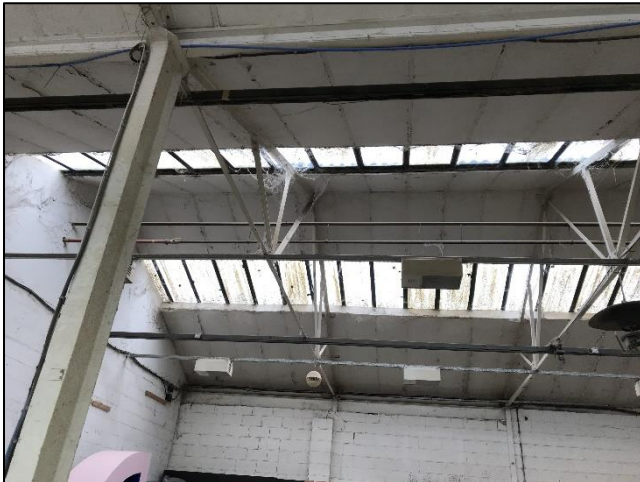
Appendix B Figure 13: Workshop roof with windows filling the unit with light
