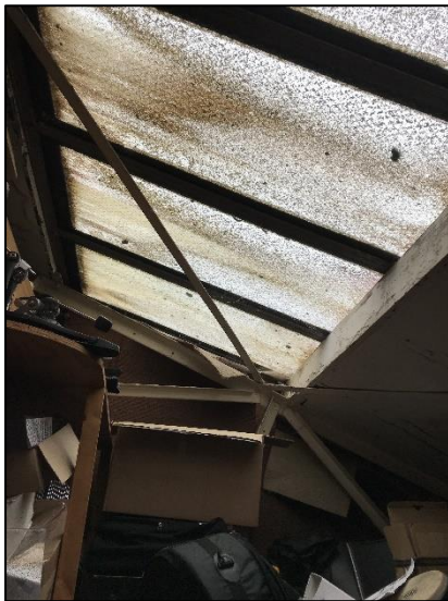
Appendix B Figure 6: Loft space window fills the loft with light
