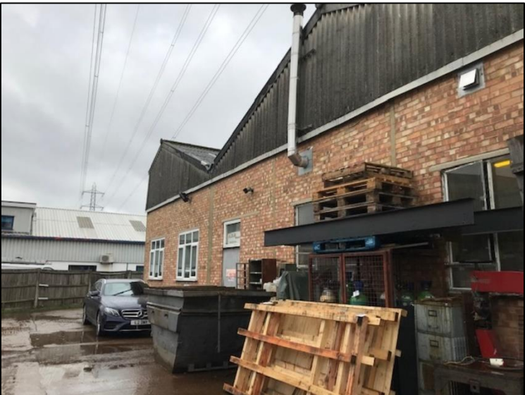
Appendix B Figure 21: Front face of Unit C facing west toward the industrial yard
