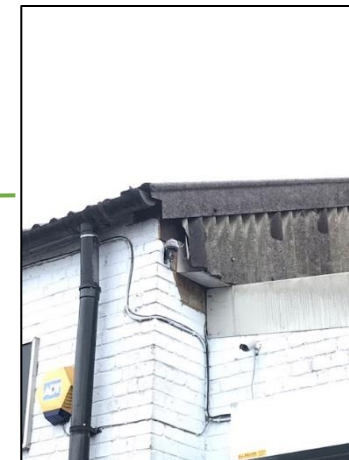
Unit D, gap between roof and wall
