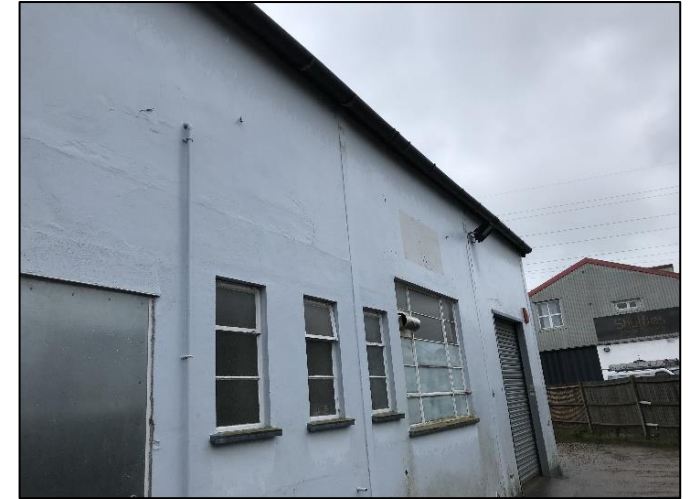
Appendix B Figure 5: Northern wall Unit A facing north
