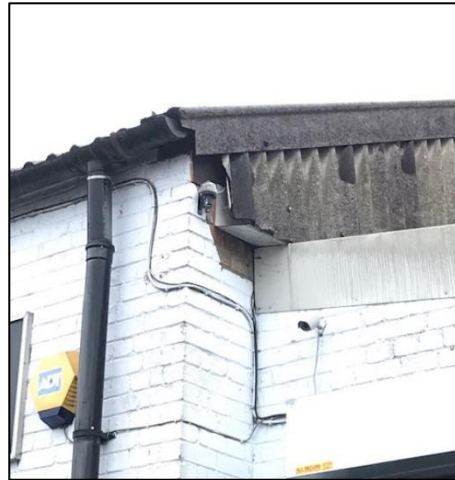
Appendix B Figure 31 : Access point between roof and wall
