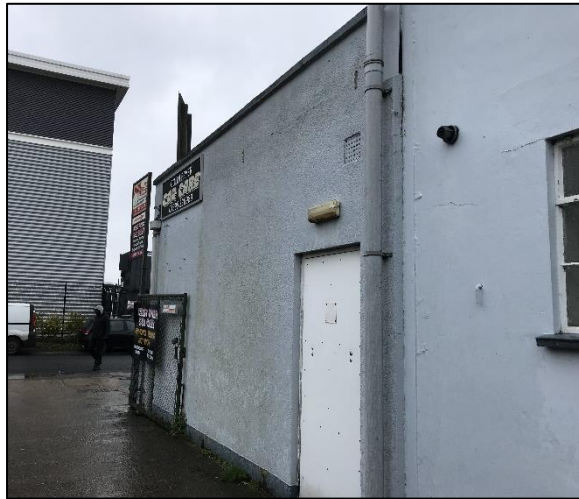
Appendix B Figure 4: Northern wall of Unit A facing north
