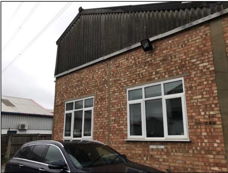
Appendix B Figure 18: Northern wall of Unit C
