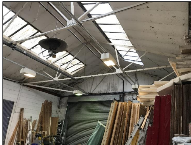
Appendix B Figure 14: Workshop roof with no ceiling cavity
