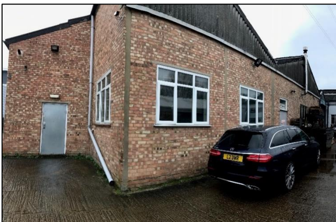
Appendix B Figure 16: Front of Unit C facing southwest
