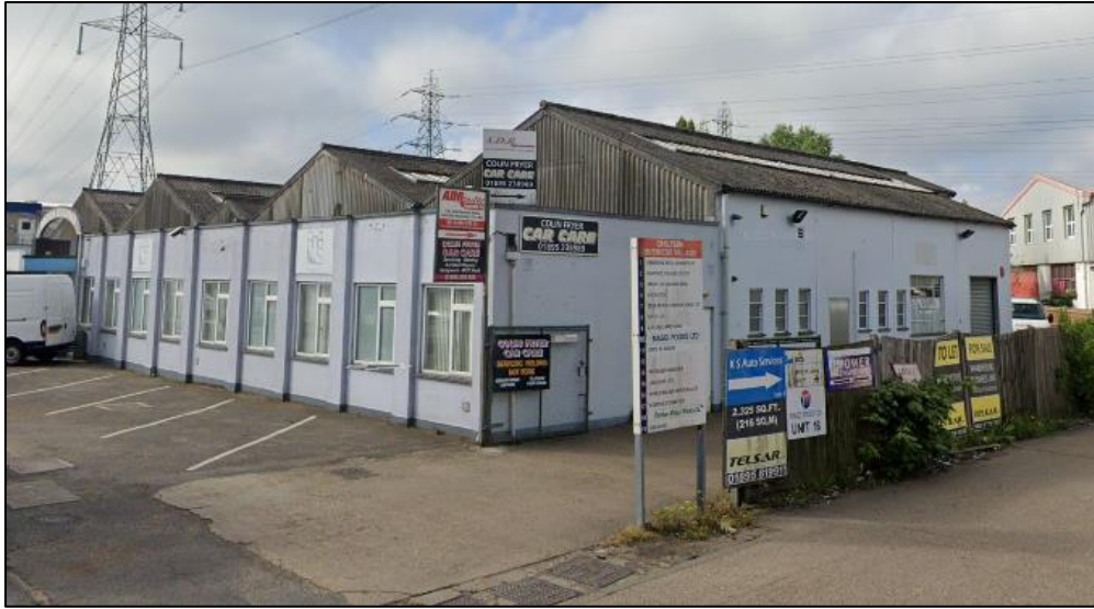
Figure 3: Barton Buildings frontage looking south west from Arundel Road (Google Street View). Arrow displaying location where photo is taken. The front building is unit A and connects to unit C behind.
