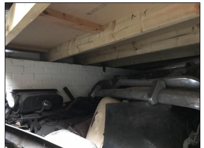
Appendix B Figure 27: Beams underneath darker Mezzanine area
