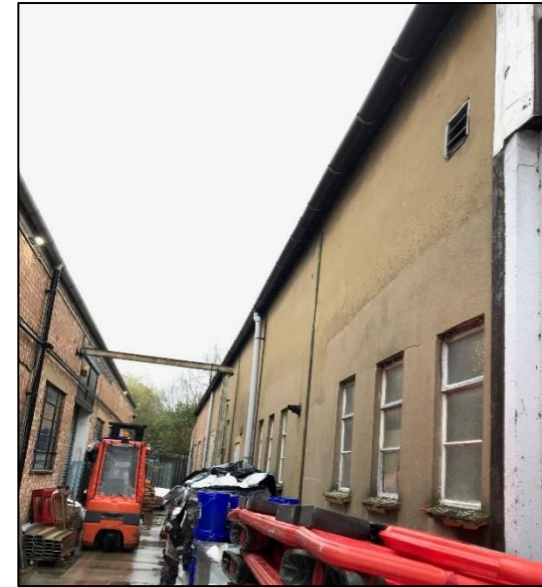
Appendix B Figure 12: Alley between adjacent buildings with a flood light
