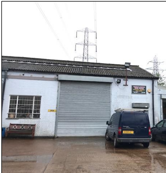
Appendix B Figure 28: Front of Unit D facing south in the building's yard
