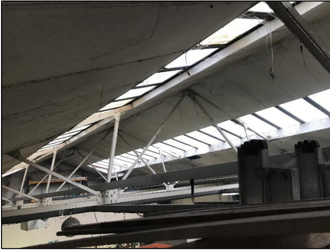
Appendix B Figure 22: Pitched roof with windows running the length of the building keep the warehouse in light
