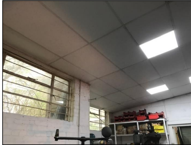
Appendix B Figure 43: Windows fill the unit with light
