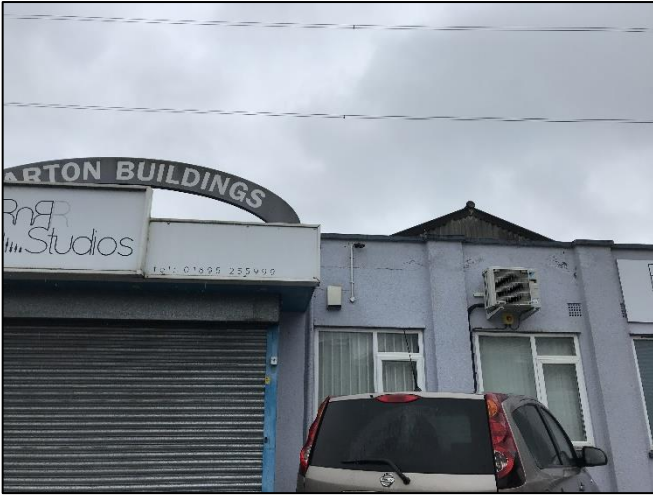
Appendix B Figure 3: Unit A front, flat concrete roof with roller door
