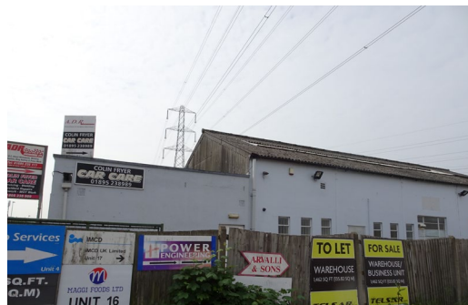
Side of building with overhead powerline shown
