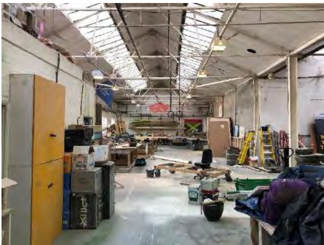
Inside Trinity building
