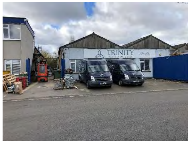
Front of Trinity works on Arundel Road
