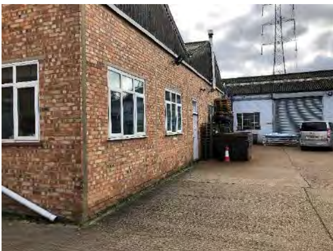
View across rear yard
