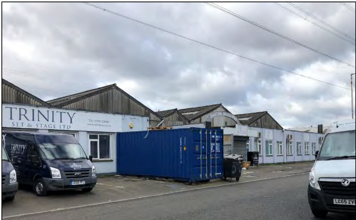
Photograph 1: View of the site from Arundel Road
